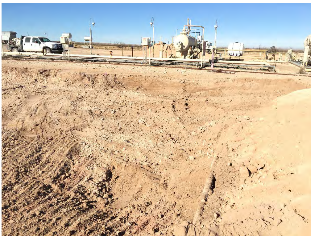
Indian Basin Station 210 – Excavation, Section B (Looking North)
