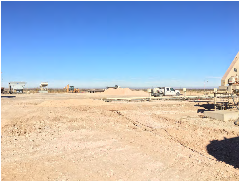
Indian Basin Station 210 – Excavation, Section A/B Boundary (Looking North)
