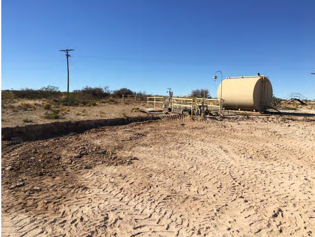
Indian Basin Station 210 - Excavation, Section A (Looking Northwest)
