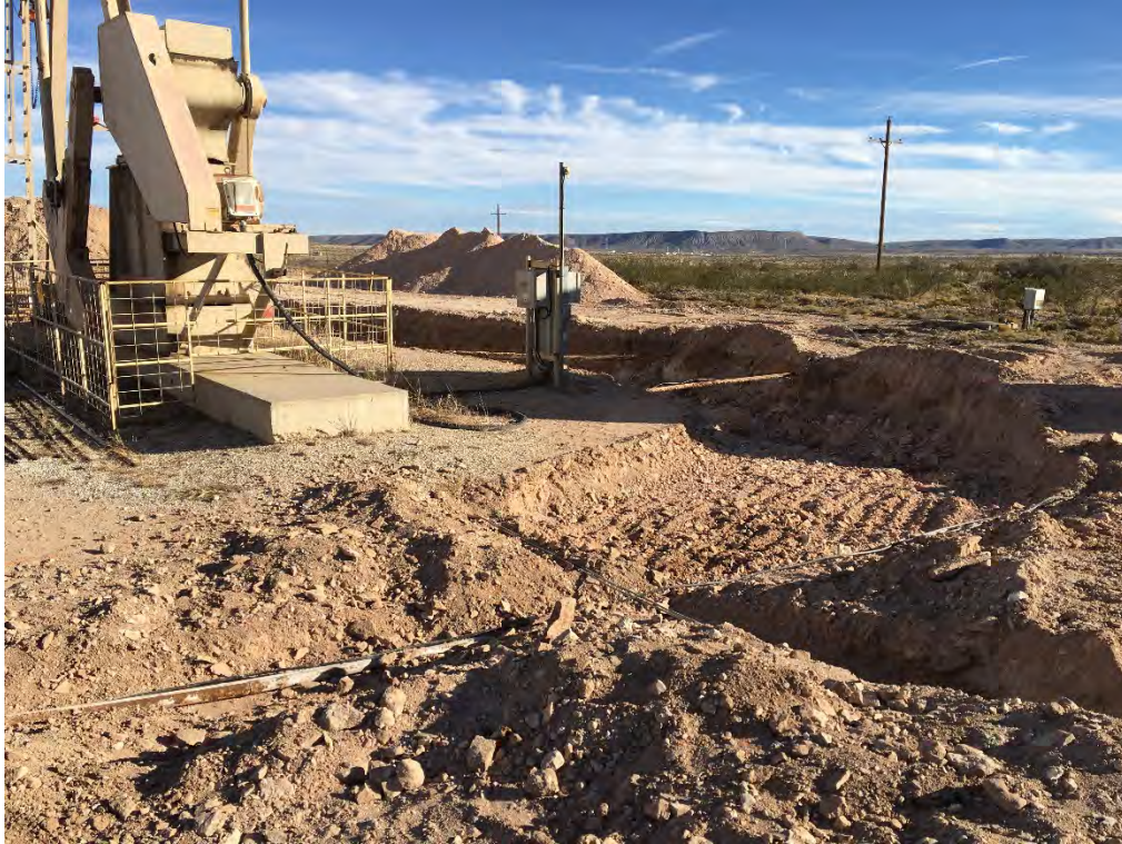
Indian Basin Station 210 – Excavation, Section B (Looking Southeast)
