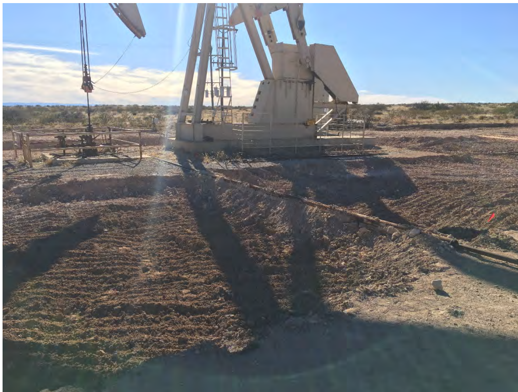
Indian Basin Station 210 - Excavation, Section B (Looking South-Southwest)
