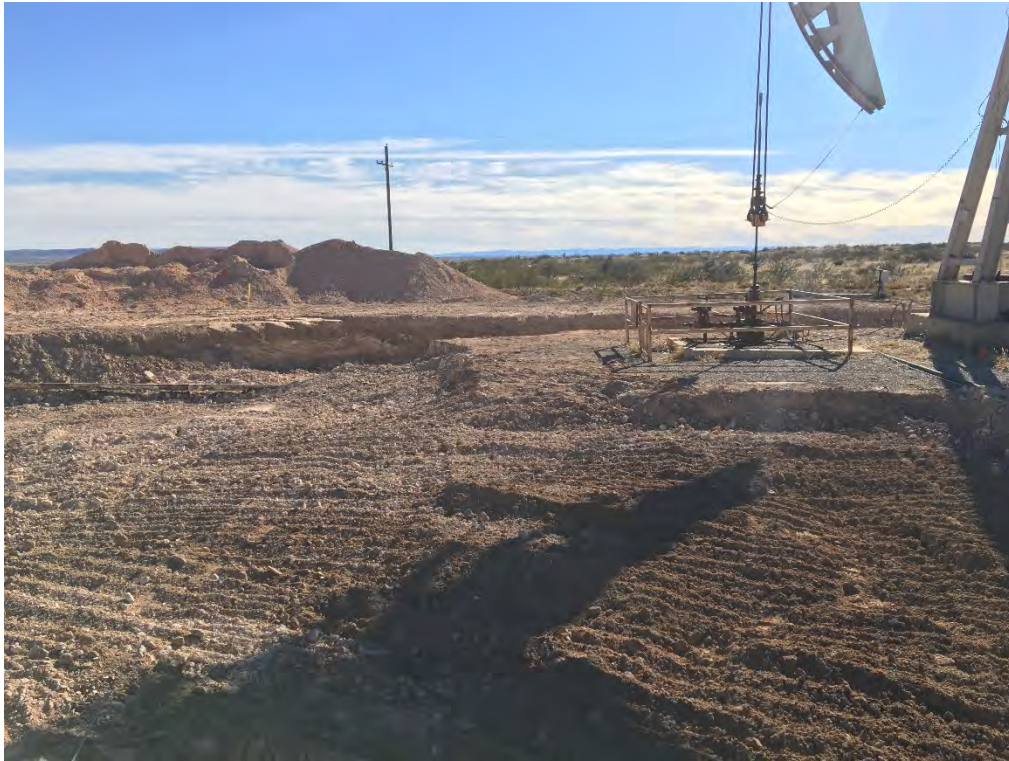
Indian Basin Station 210 - Excavation, Section B (Looking South)
