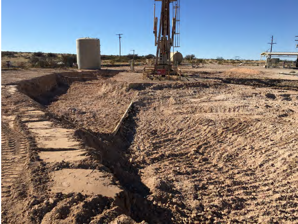
Indian Basin Station 210 - Excavation, Section B (Looking West)
