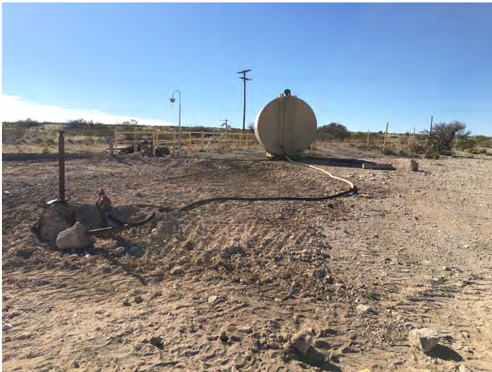
Indian Basin Station 210 – Excavation, Section A (Looking West)
