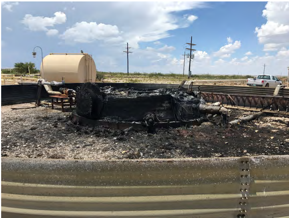
Indian Basin Station 210 - Release (Looking Northwest)
