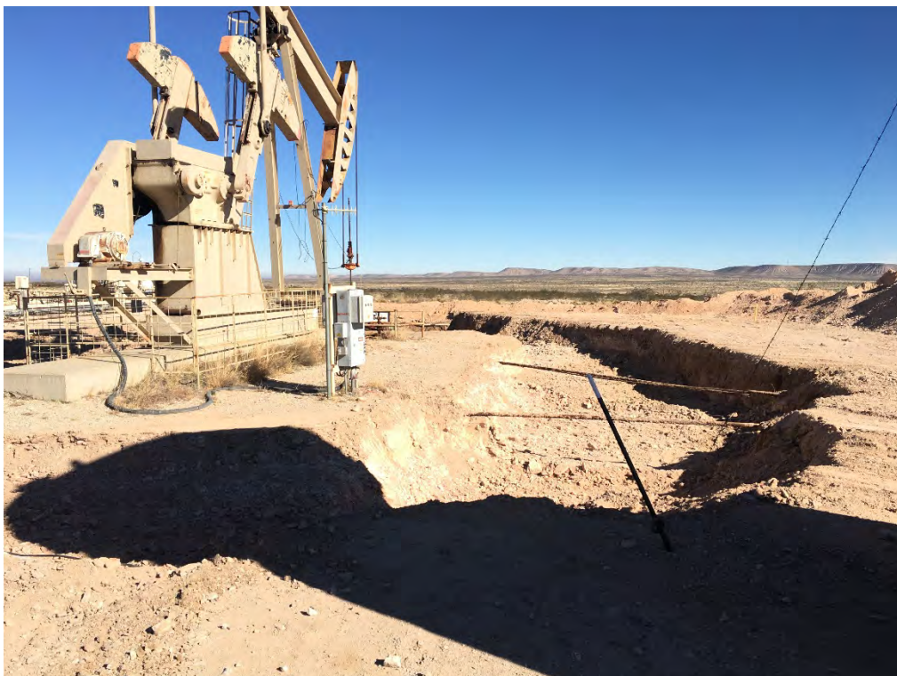
Indian Basin Station 210 - Excavation, Section B (Looking East-Northeast)
