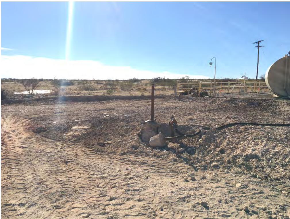
Indian Basin Station 210 - Excavation, Section A (Looking Southwest)
