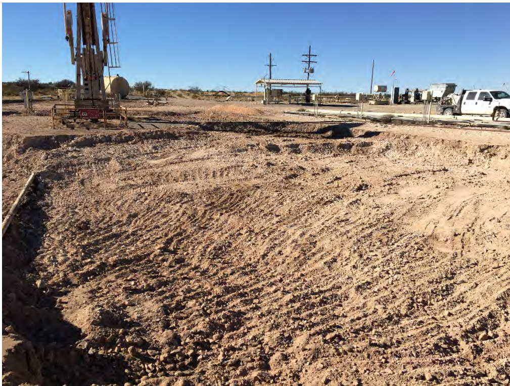
Indian Basin Station 210 – Excavation, Section B (Looking West-Northwest)
