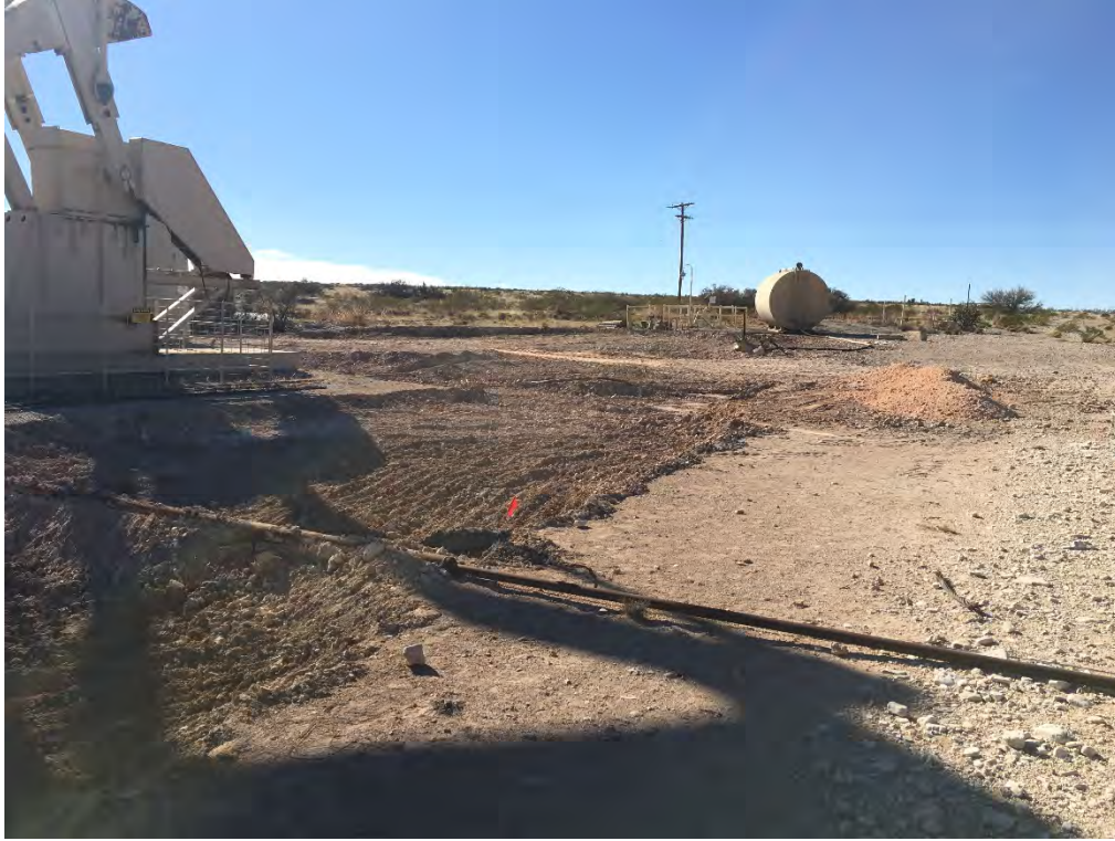
Indian Basin Station 210 – Excavation, Section B (Looking East-Southeast to Section A)
