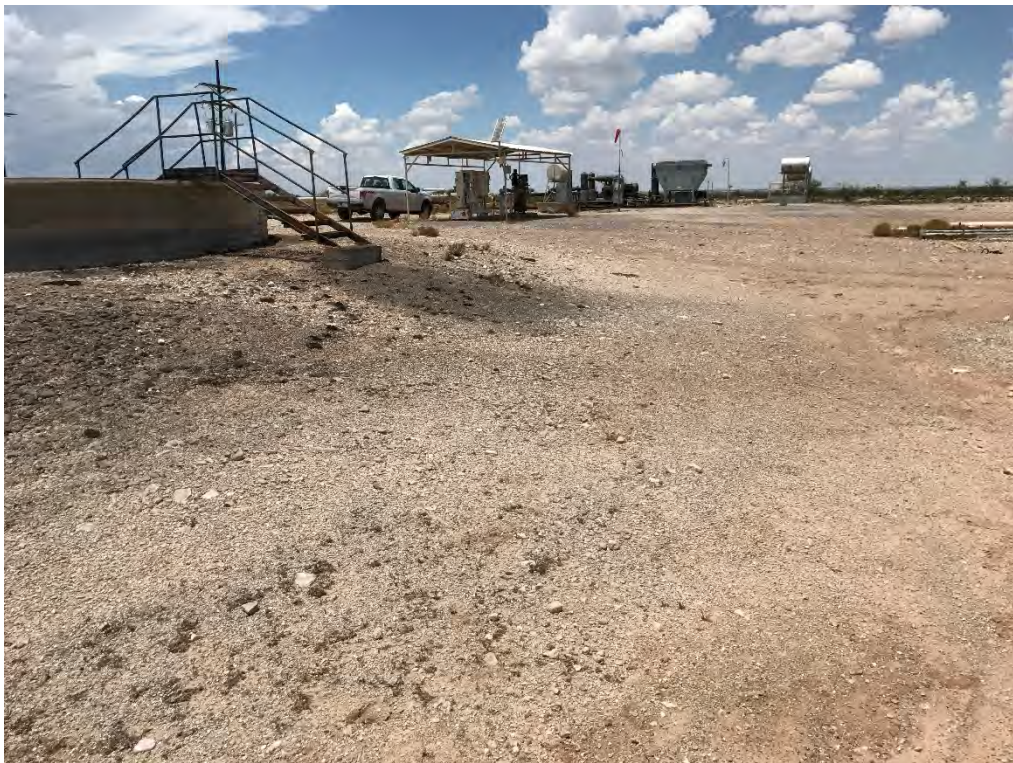
Indian Basin Station 210 – Release (Looking Northwest)
