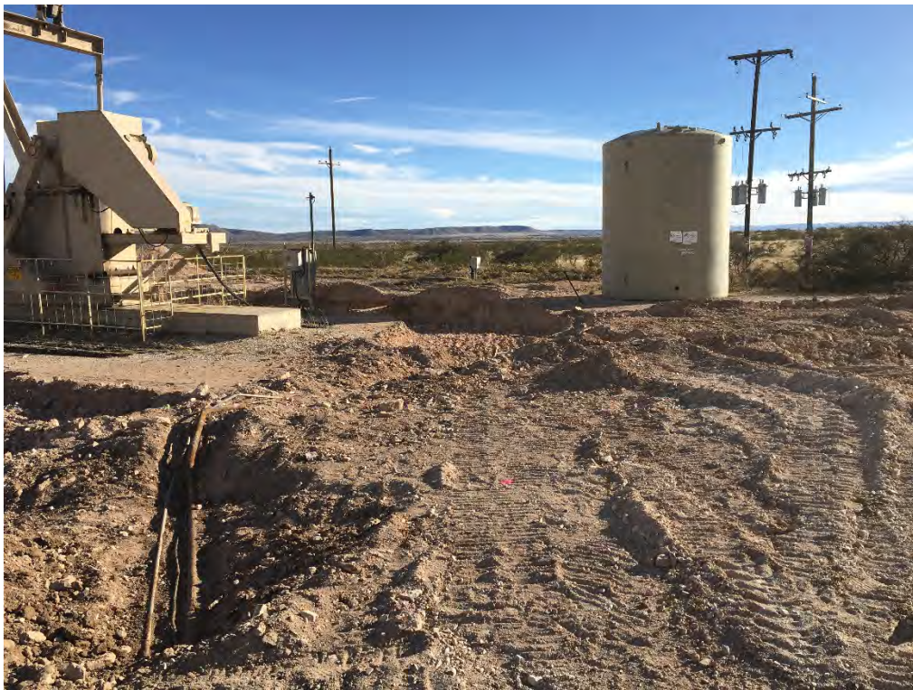
Indian Basin Station 210 - Excavation, Section B (Looking South-Southeast)
