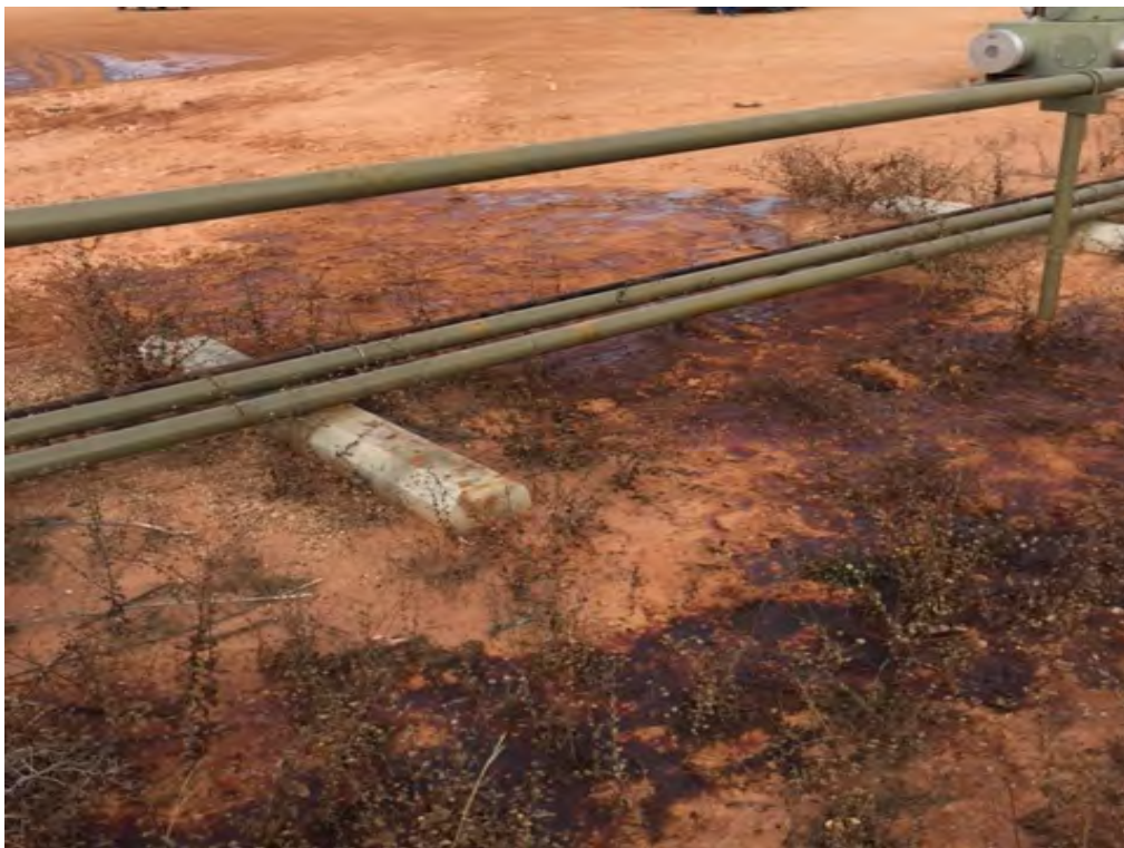
Federal 12 #14H – Release (Looking Northwest)
