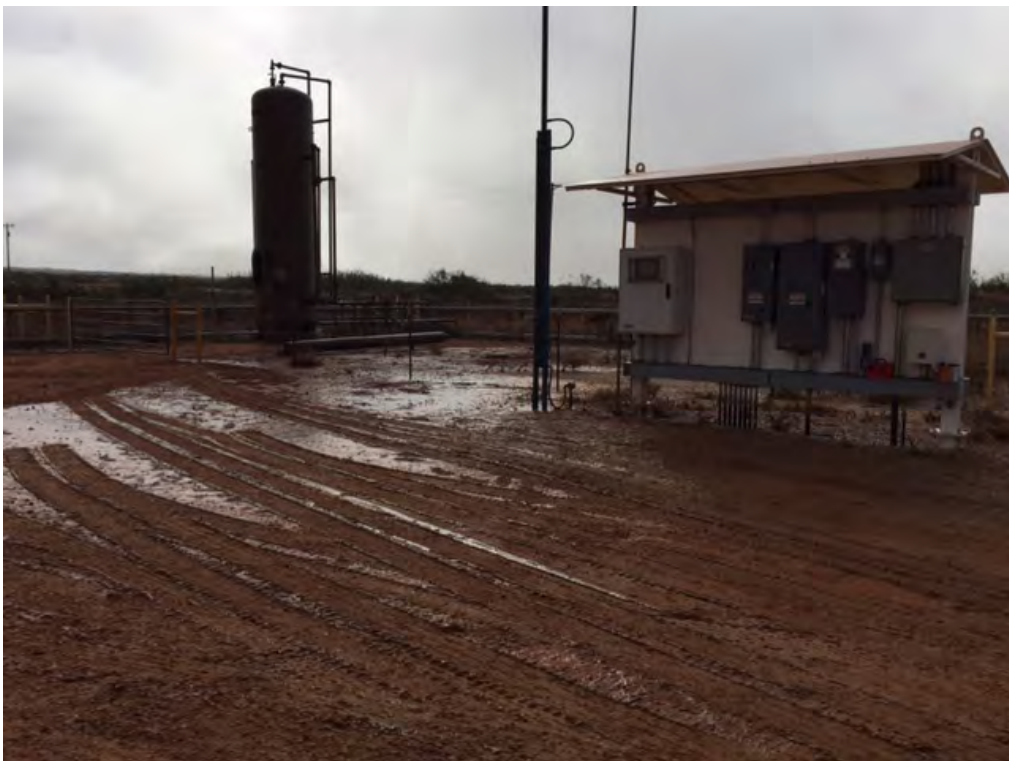
Federal 12 #14H – Release (Looking Southeast)
