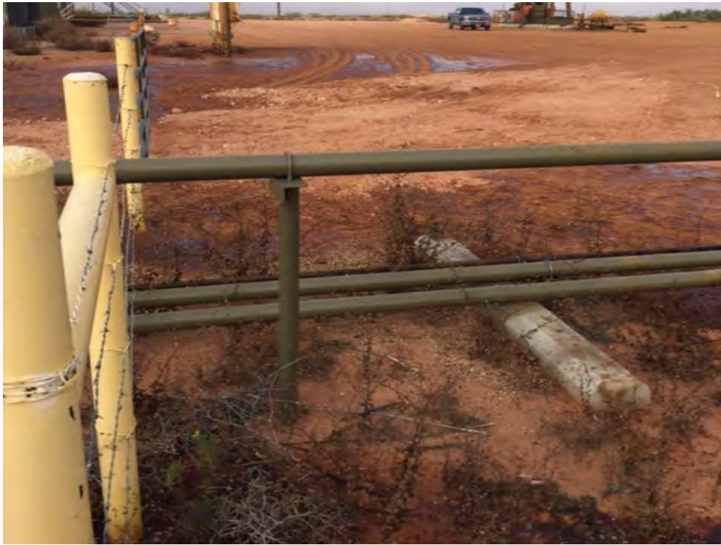
Federal 12 #14H – Release (Looking West-Northwest)
