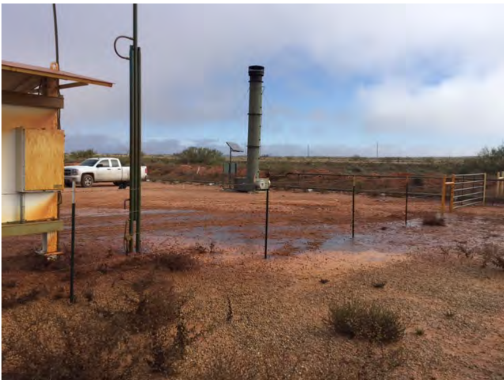
Federal 12 #14H – Release (Looking Northeast)
