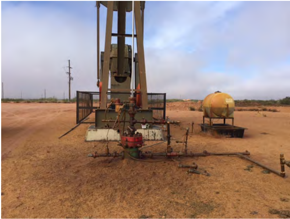
Federal 12 #14H – Overspray Area (Looking West)
