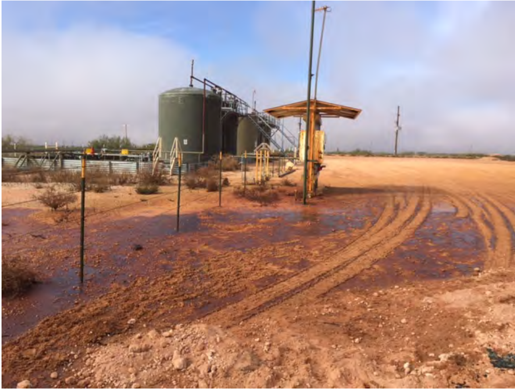
Federal 12 #14H – Release (Looking West)
