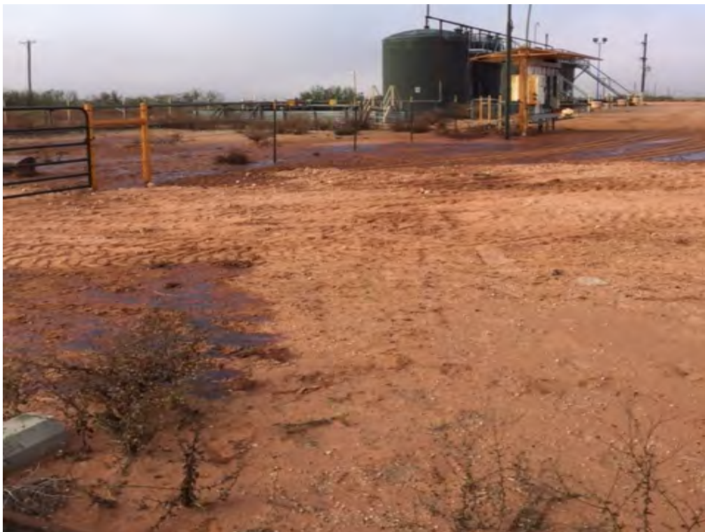
Federal 12 #14H – Release (Looking West-Southwest)
