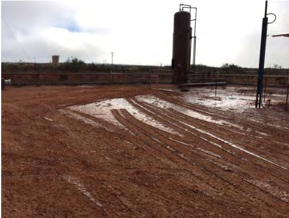
Federal 12 #14H – Release (Looking Southeast)
