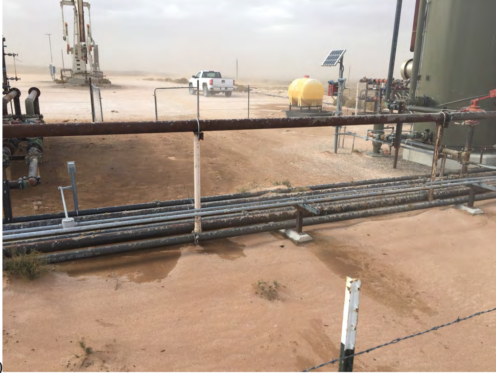
FNR 26 1 CTB – Release (Looking West-Northwest)
