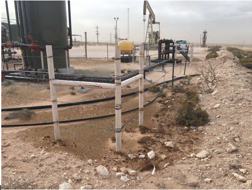
FNR 26 1 CTB – Release (Looking Southwest)
