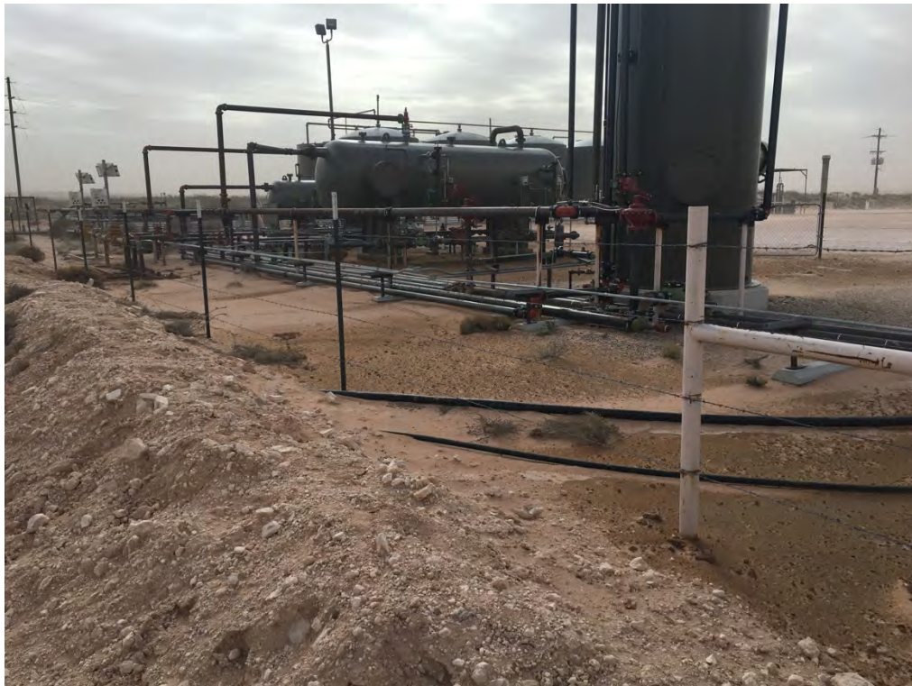
FNR 26 1 CTB – Release (Looking Southwest)
