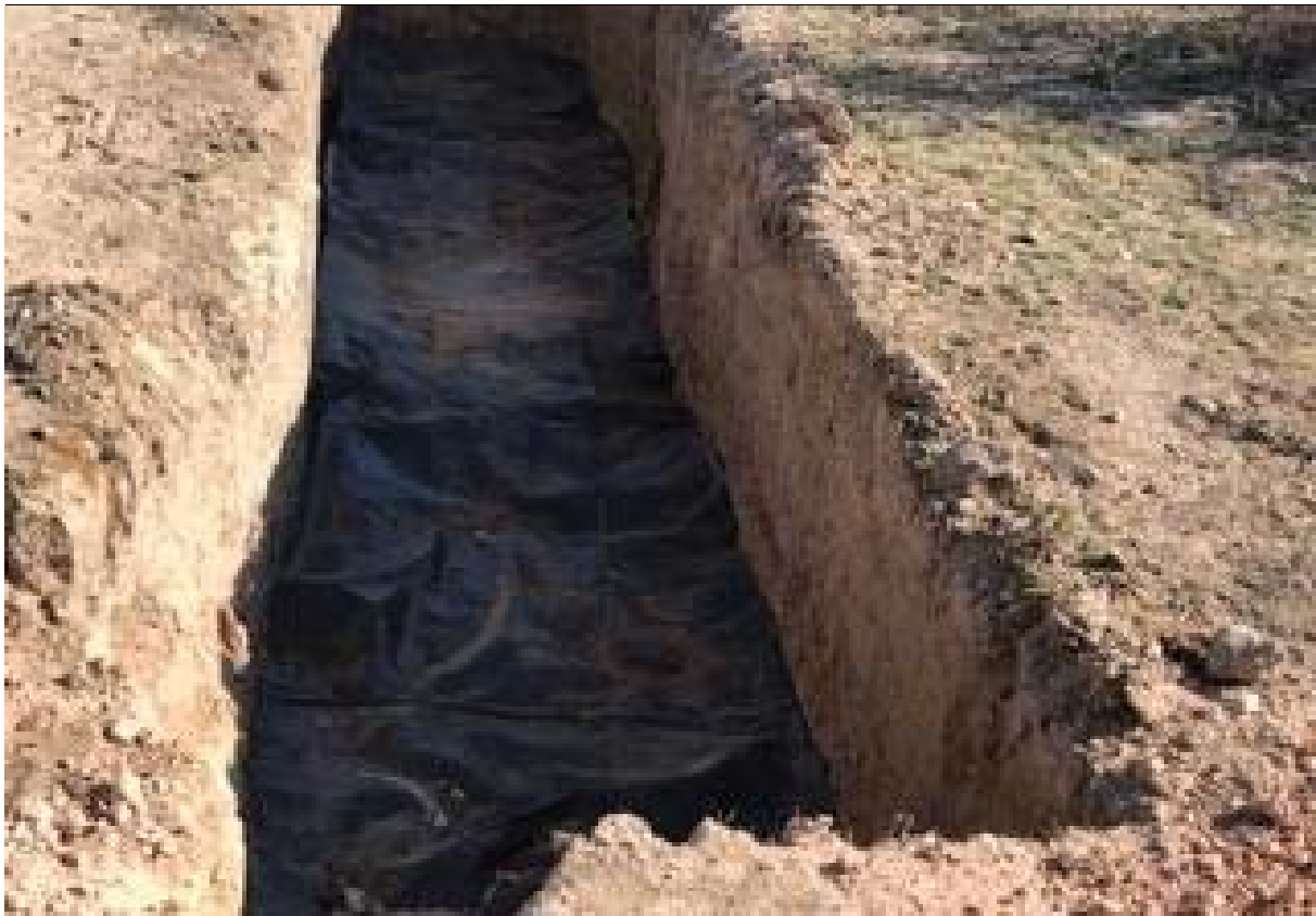
Figure 9 - View of portion of the excavated area and liner installation.
