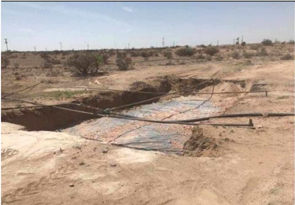
Figure 8 - View of portion of the excavated area and liner installation.
