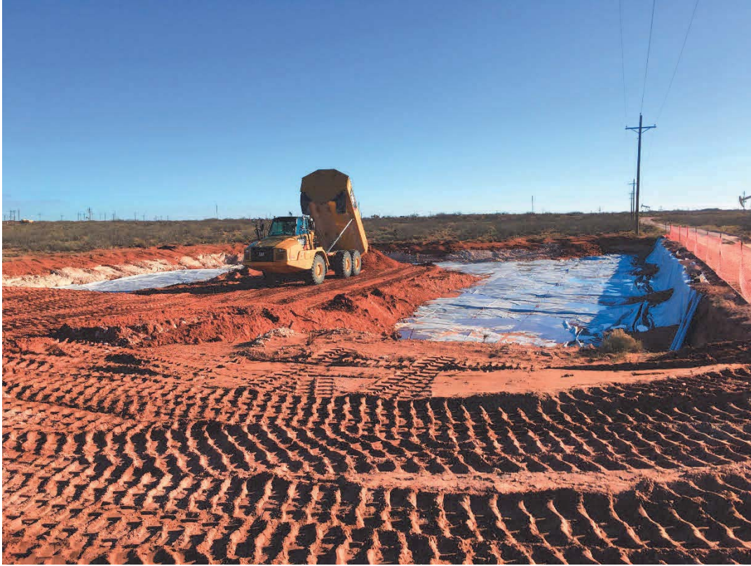
Figure 1: Cross sectional view of backfill with poly liner in place in Area A
