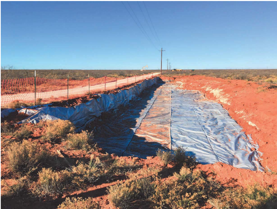
Figure 2: Poly liner shown in place in Area B.
