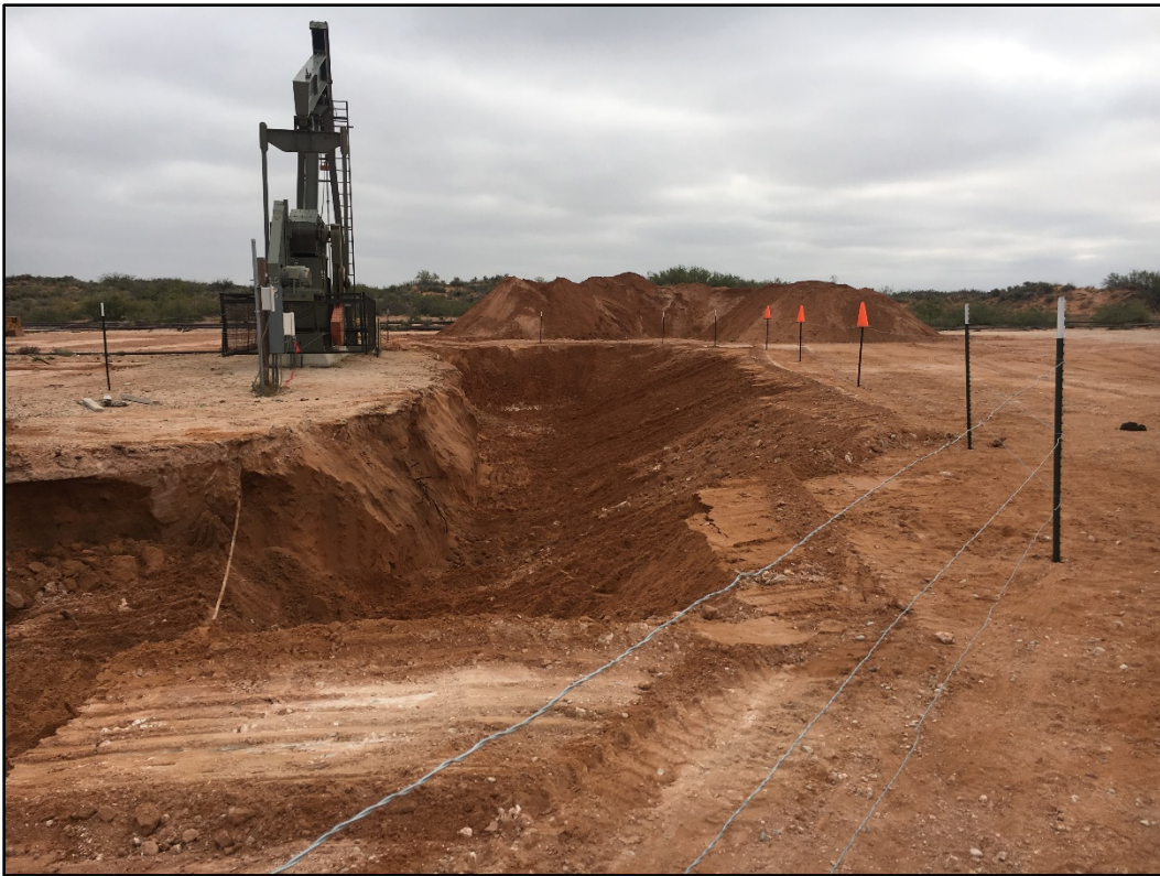
Photo 9. Excavation secured using 3-wire fencing.
