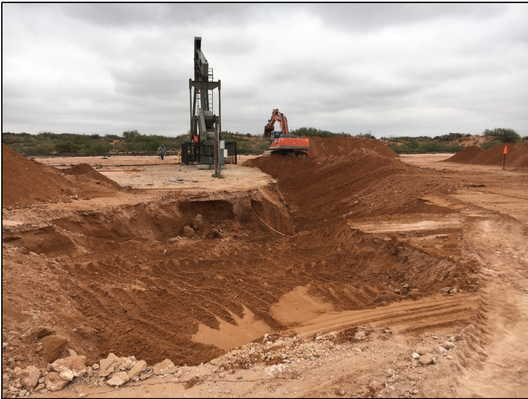
Photo 6. Excavation activities. Note exposed electrical line in center of photo.
