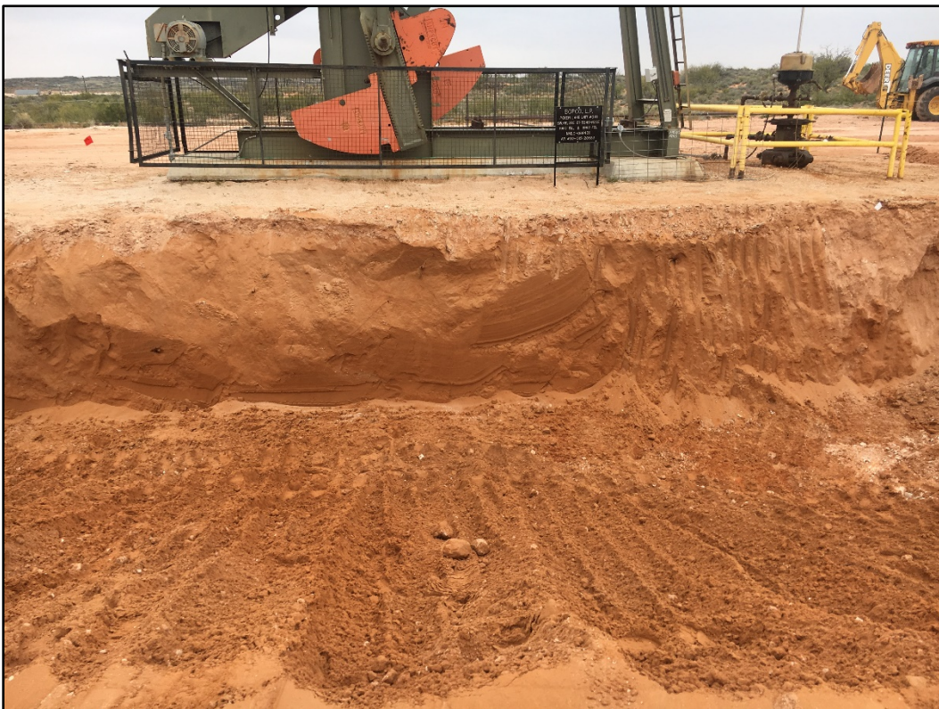
Photo 8. Scraping the walls for samples SC-12 and SC-13.
