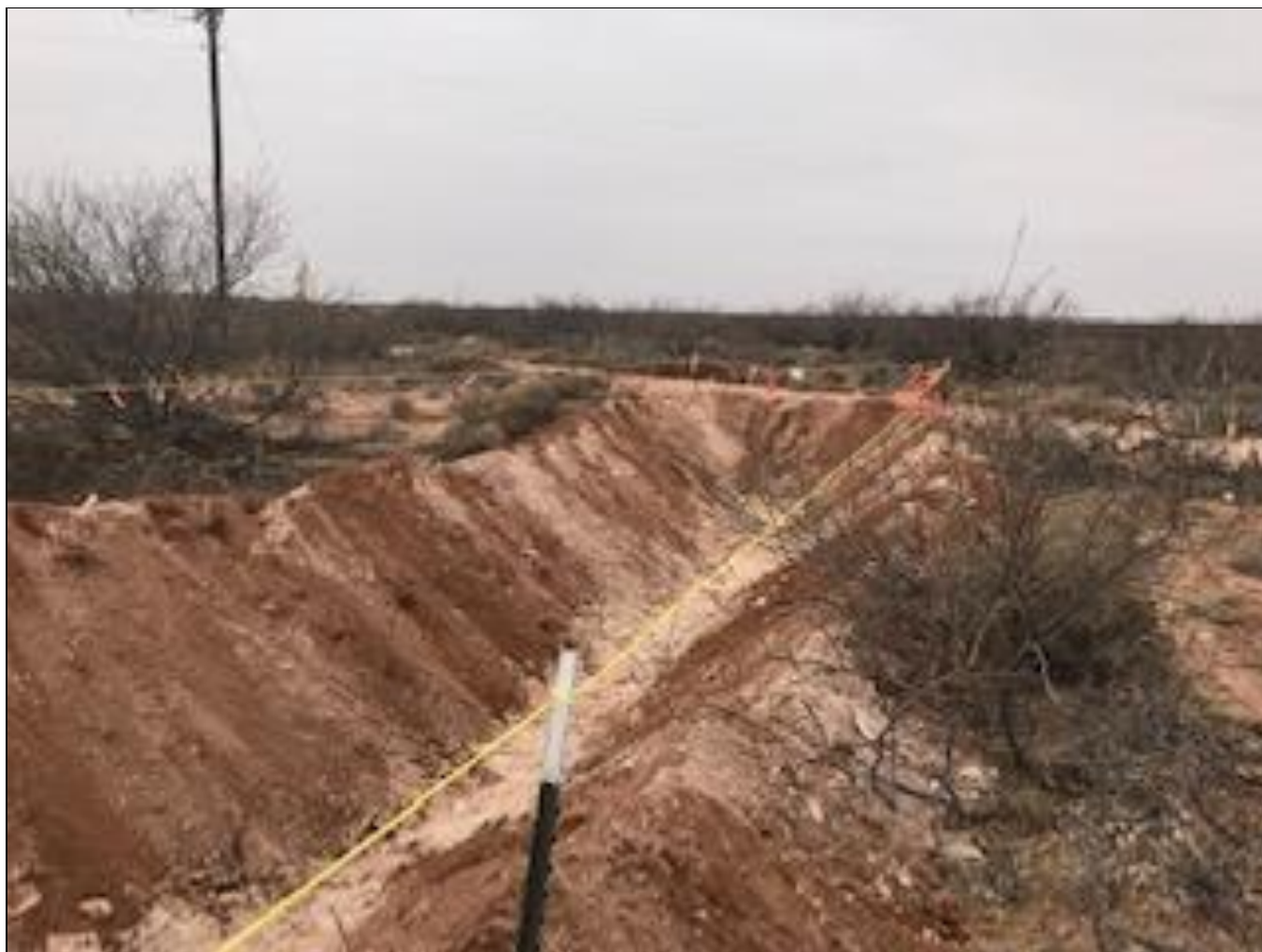
View of excavation from the north edge of the well pad facing south.
