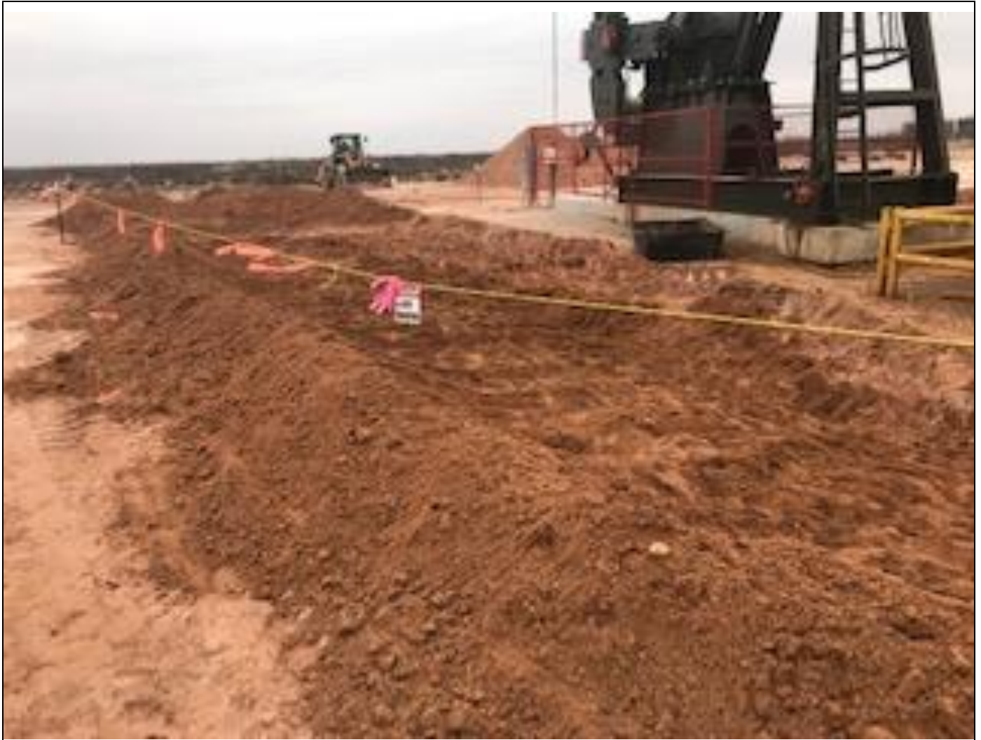
View of excavation on well pad from pumpjack facing north.
