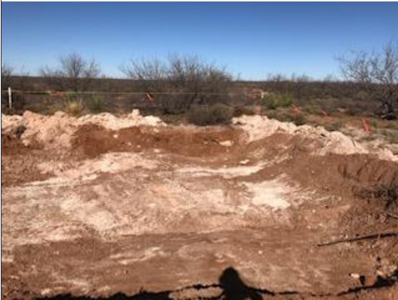
View facing north of pasture excavation north of the road.
