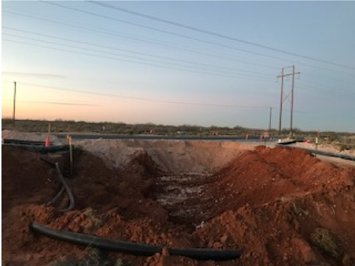
North facing view facing of the excavation.
