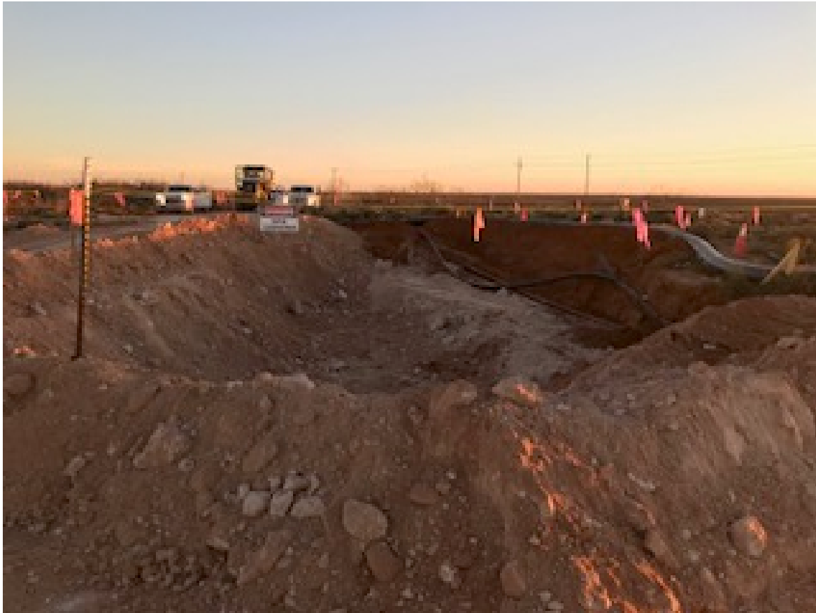
Southwest facing view facing of the excavation.
