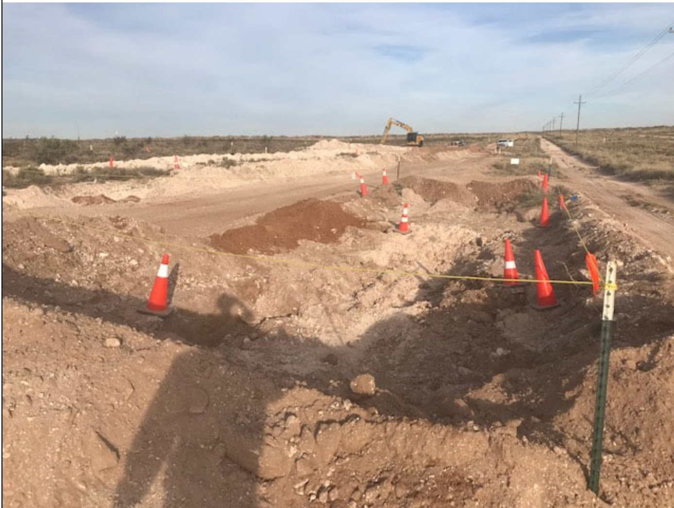
View east between the right-of-way showing excavation.
