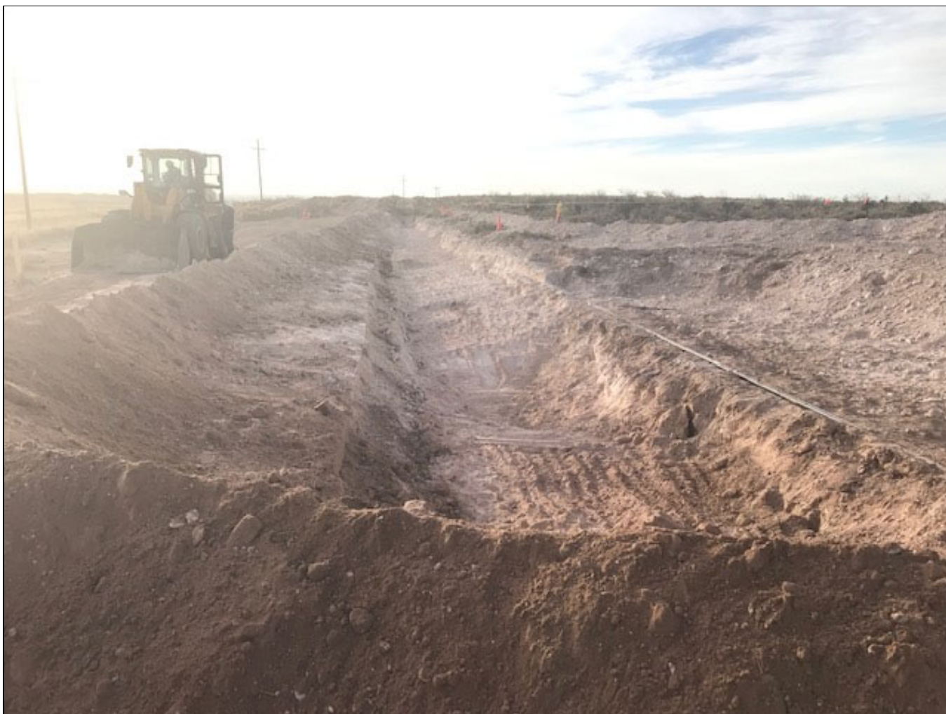
View west of the excavation.
