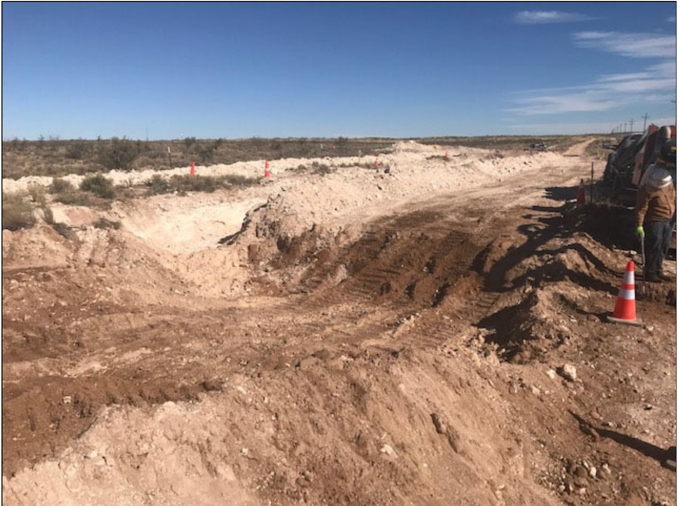
View east of the excavation between the pipelines.
