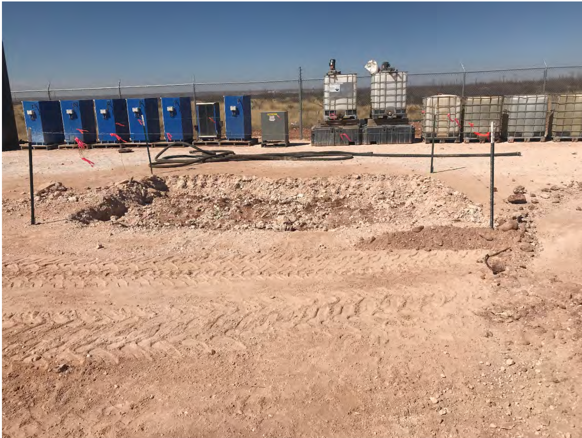
View northwest of the open excavation.
