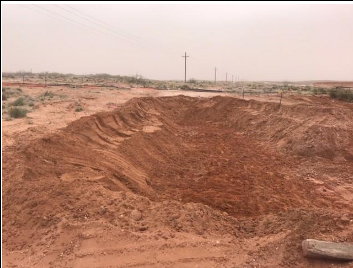
Eastern view of final excavation extent.
