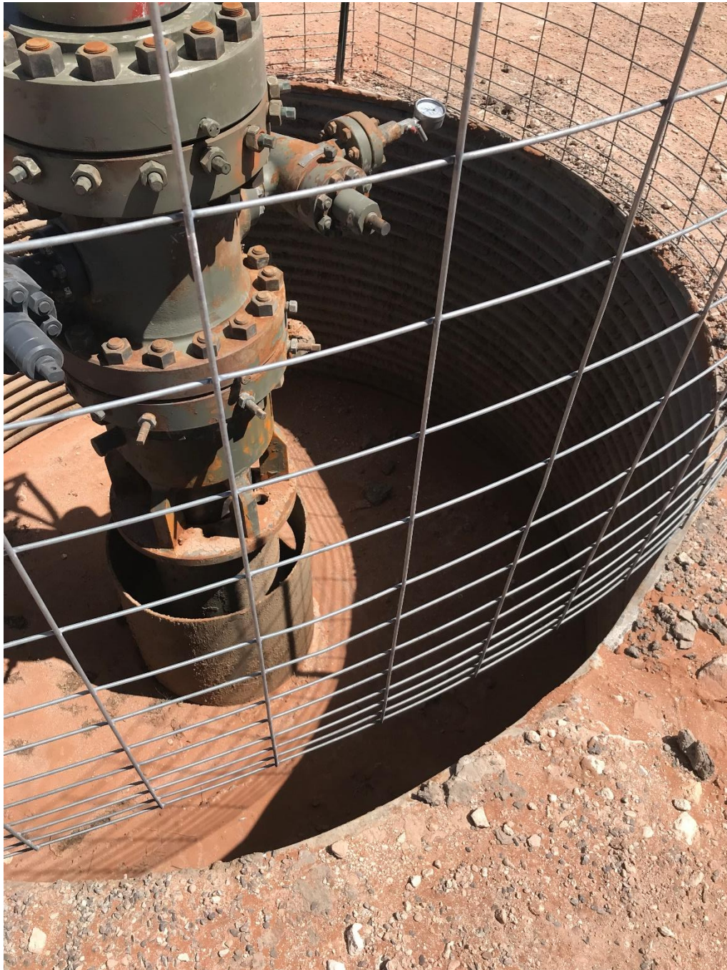
Closeup view of point of release and well cellar.
