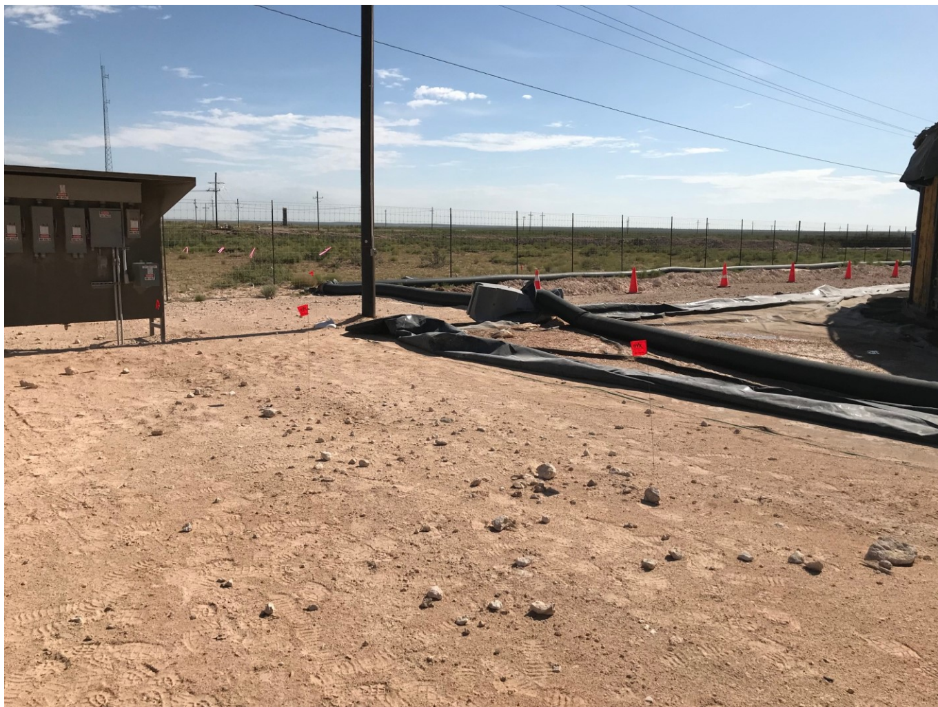
Northeastern view of the active pipelines area after the excavation was backfilled.
