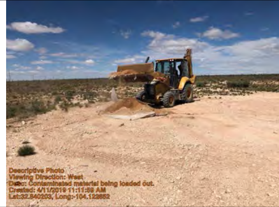
Contaminated material being loaded out.
