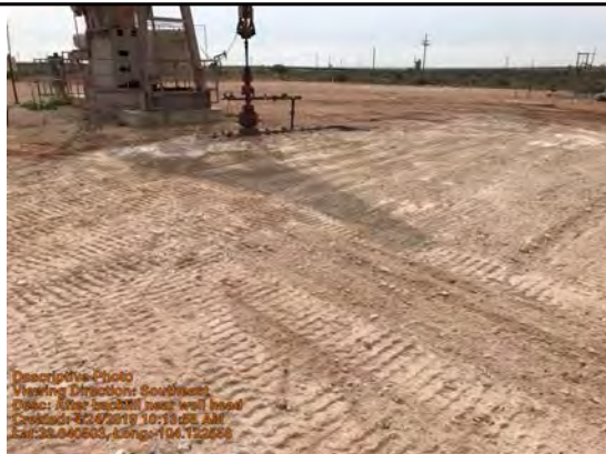
After backfill near well head
