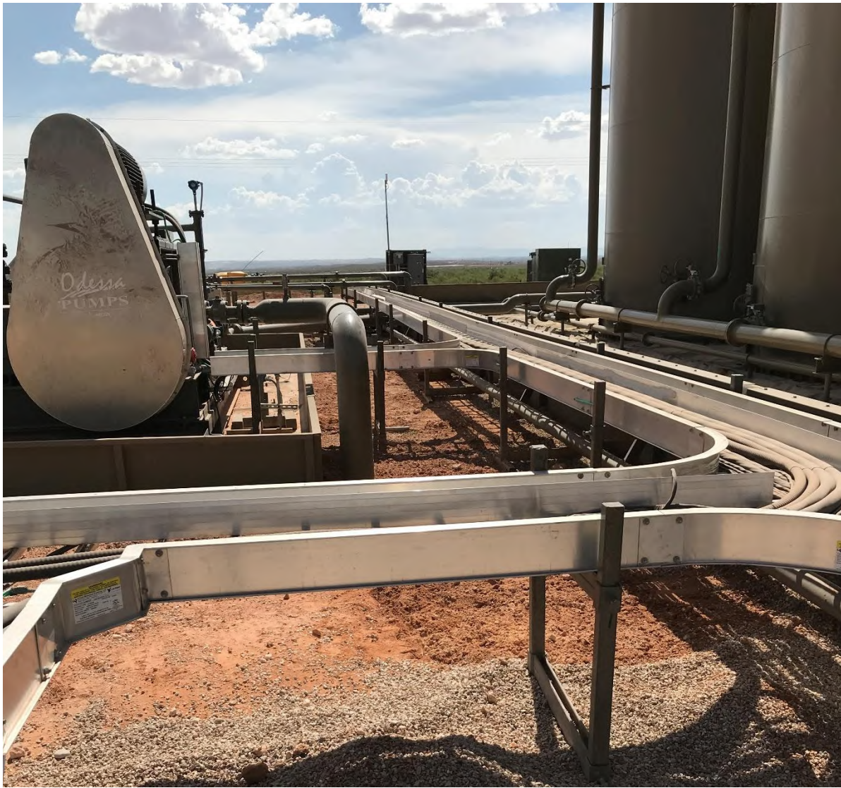
Western view of final excavation extent.
