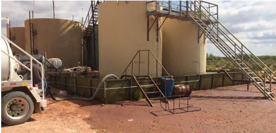
Figure 3: Tank battery where the release overflowed along the southern end of the containment wall. Stained soil is the release. Photo is viewing northeast. Date/Time: 2019-06-12 09:40:51. GPS: 32.4335889 N , -103.6174389 W
