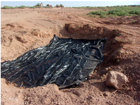
Backfilled to 4' - lined
