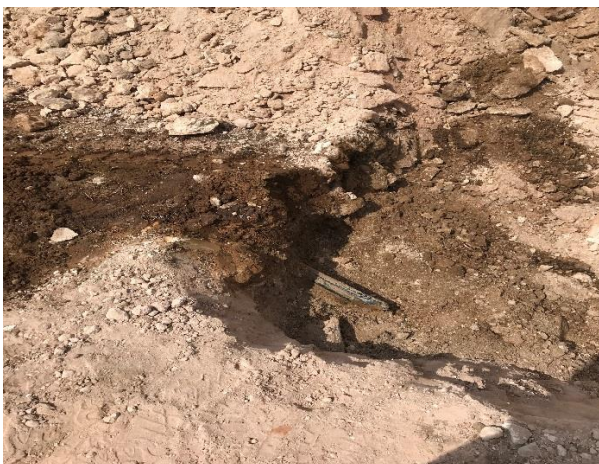
Line Strike in Test Trench
