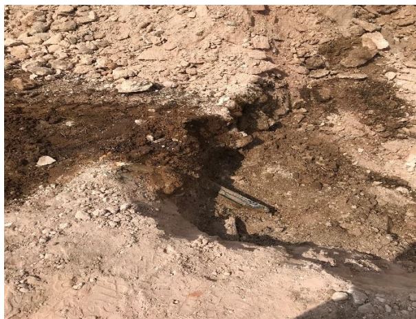
Line Strike in Test Trench
