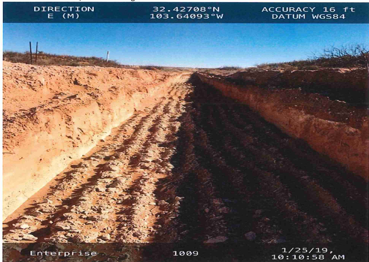
Excavation Flow Paths, Note Benching Side Walls
