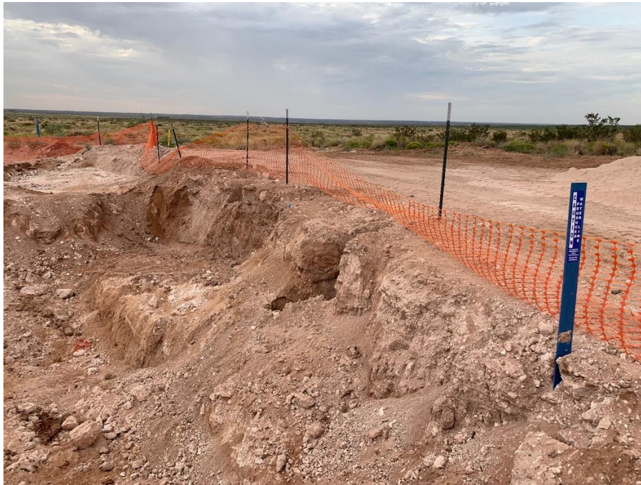
Photo 17: Off Right of Way Excavation – looking SE at south wall
