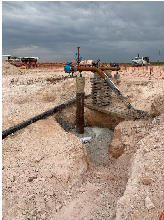
Photo 8: Main Excavation – new sono column (TD = 16ft)
