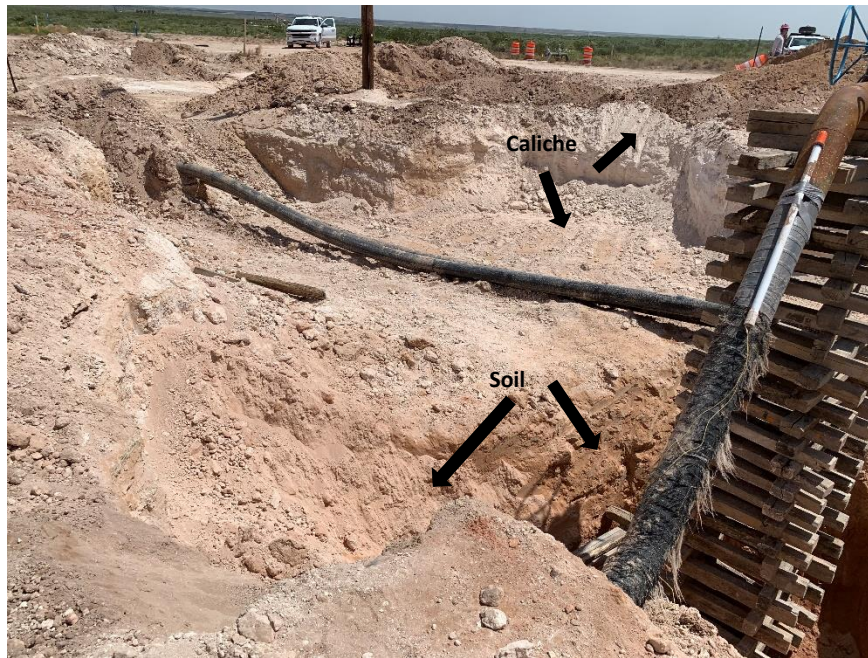
Photo 7: Main Excavation— heterogeneous subsurface caliche and soil
