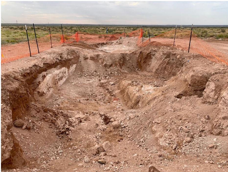
Photo 18: Off Right of Way Excavation – looking SE at final excavation area
