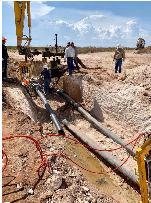
Photo 3: Main Excavation Pipeline Repair
