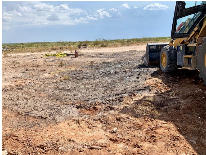
Photo 2: Burnt Area from Electrical Fire – looking South
