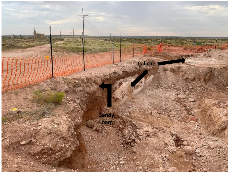
Photo 15: Off Right of Way Excavation – looking East – heterogeneous material north wall
