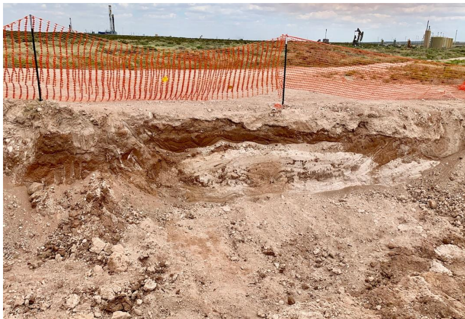
Photo 16: Off Right of Way Excavation – looking North – heterogeneous material north wall
