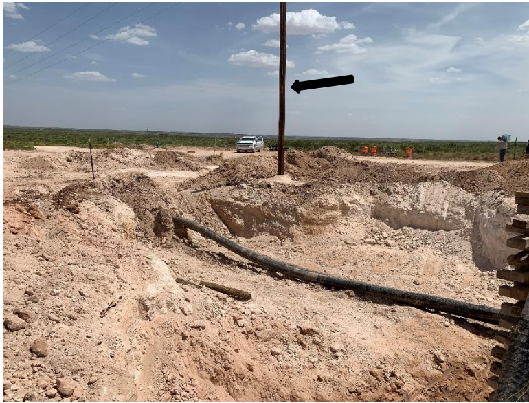
Photo 5: Main Excavation – looking SE toward new electrical pole
