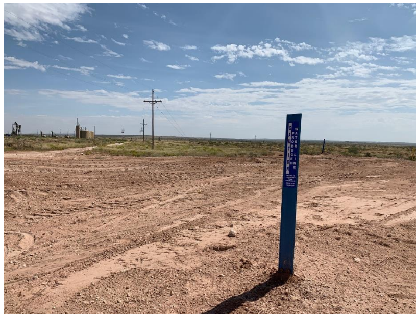
Photo 20: Off Right of Way Surface Restoration – looking SE
