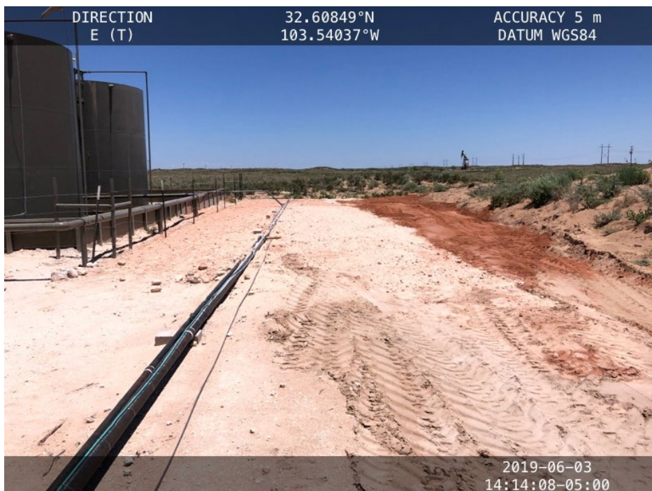
Back Filled Excavation
