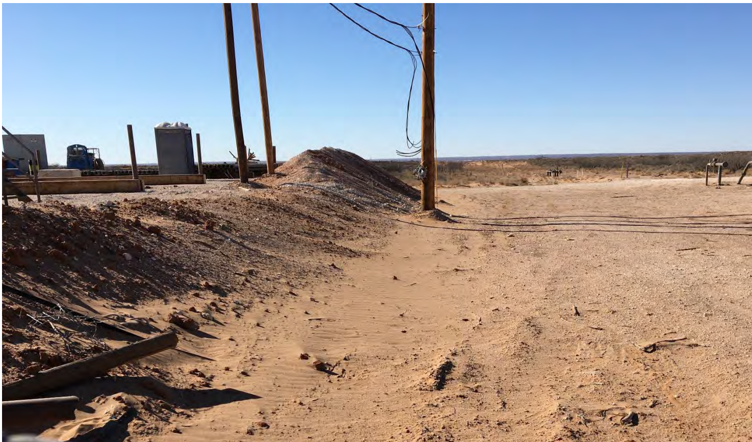
Figure 3 - View south to SW corner of pad showing lease road and in background stabilized dunes and buried pipeline. South side of pad is built in "fill".
