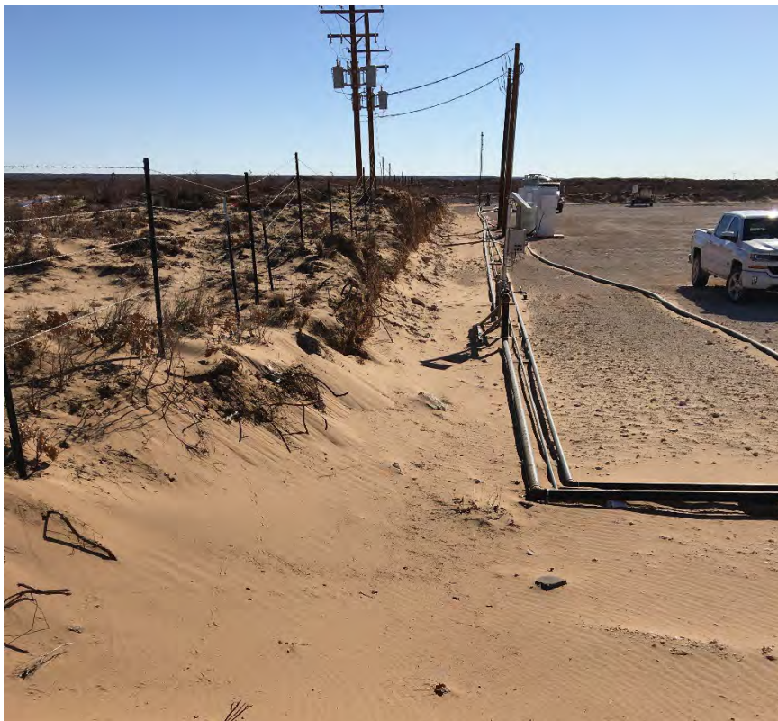
Figure 1- View east from NW corner of pad showing 1-4 foot high stabilized dunes. North side of pad is in the "cut".
