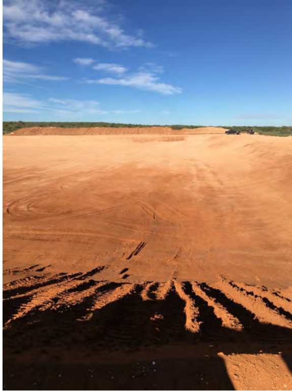
View to the west across containment excavation. Interior walls lower than required 2:1 slope
