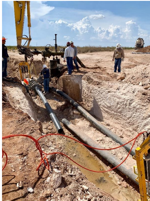
Photo 3: Main Excavation Pipeline Repair
