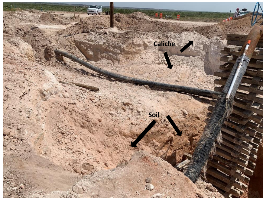
Photo 7: Main Excavation– heterogeneous subsurface caliche and soil
