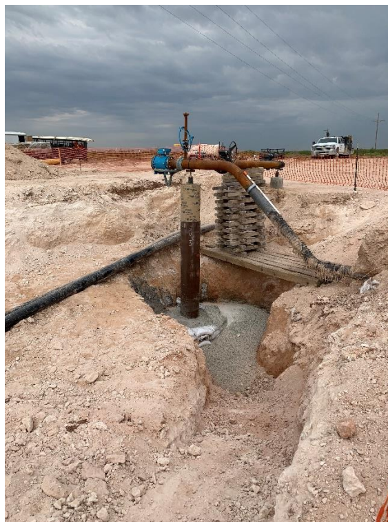
Photo 8: Main Excavation – new sono column (TD = 16ft)
