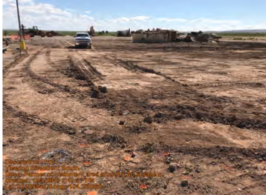
Former containment area after 0.5' scrape off
