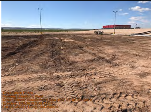
Former containment area after 0.5' scrape off
