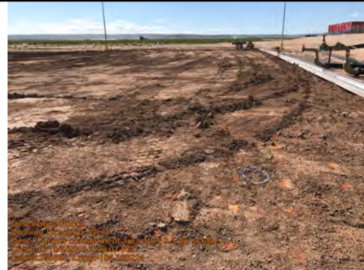
Former containment area after 0.5' scrape off
