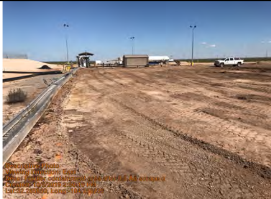
Former containment area after 0.5' scrape off
