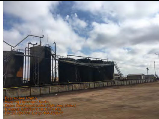
Destroyed tanks (lightning strike)
