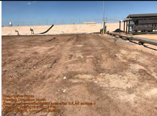
Former containment area after 0.5' scrape off
