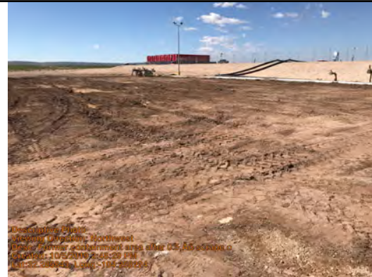
Former containment area after 0.5' scrape off
