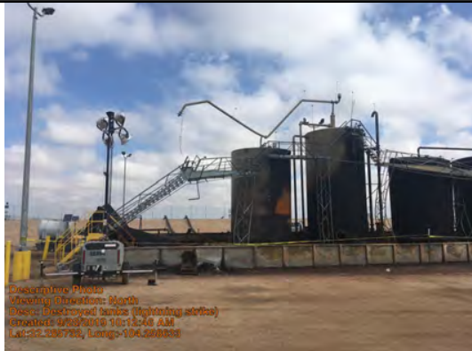
Destroyed tanks (lightning strike)
