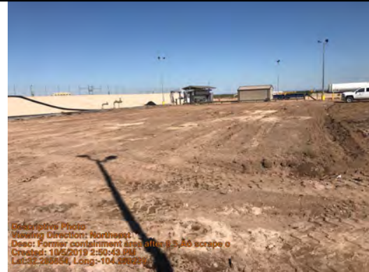
Former containment area after 0.5' scrape off
