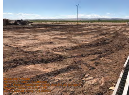
Former containment area after 0.5' scrape off
