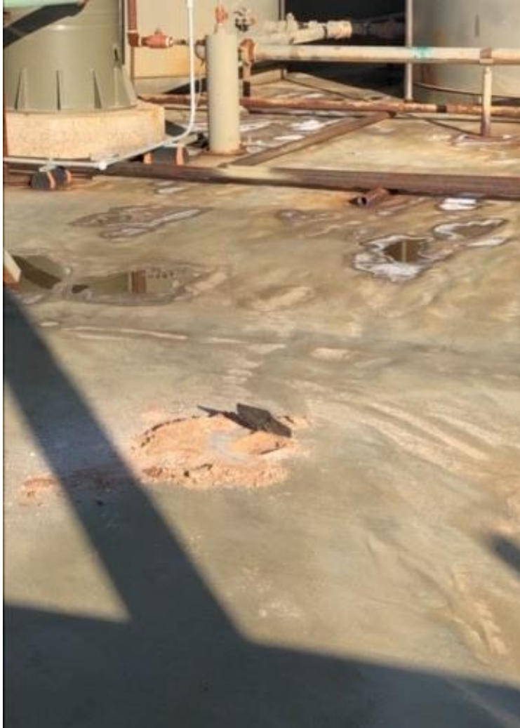
Southeastern view of lined tank battery containment and liner hole during soil sampling activities.
