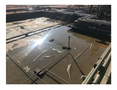
Photo 2 View of liner after repair following rain event.
