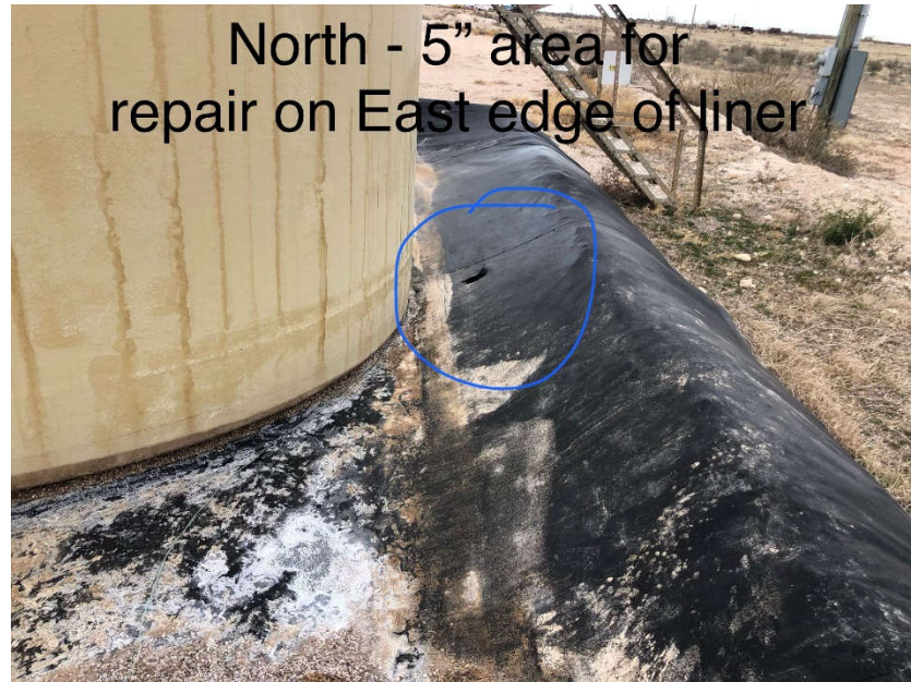
Photo 11. Location of 5-inch hole in liner on East edge of liner
