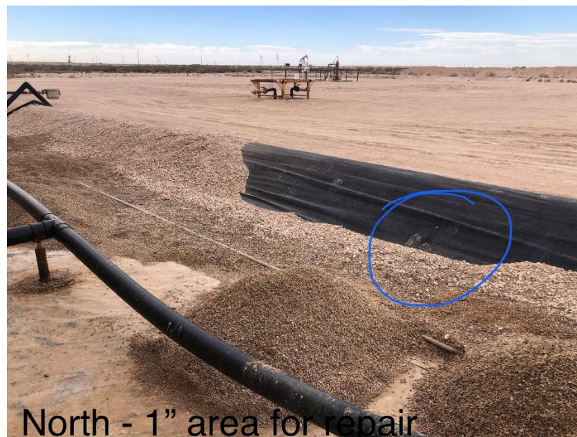
Photo 14. Location of 1-inch tears in liner on North edge of liner
