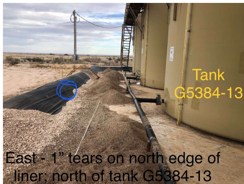
Photo 16. Location of 1-inch tears in liner on North edge of liner
