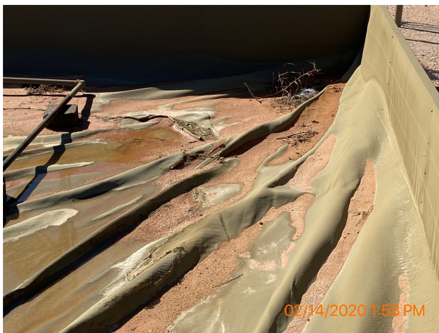
View of sediment buildup within lined secondary containment
