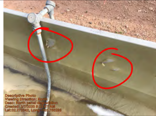
North panel degradation
