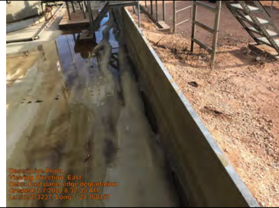
East panel edge degradation
