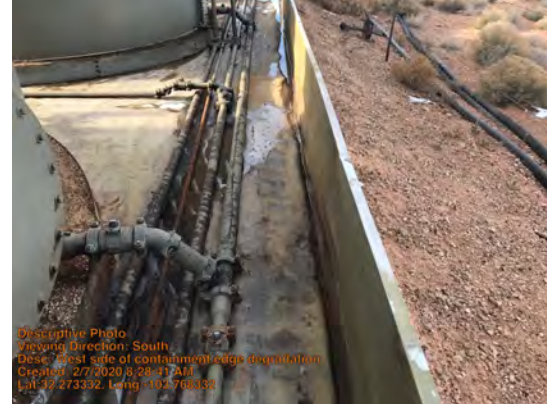
West side of containment edge degradation
