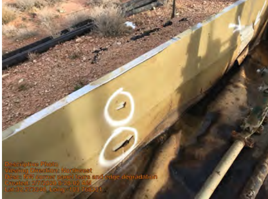
NW corner panel tears and edge degradation
