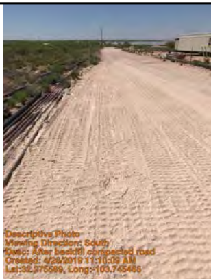
After backfill compacted road
