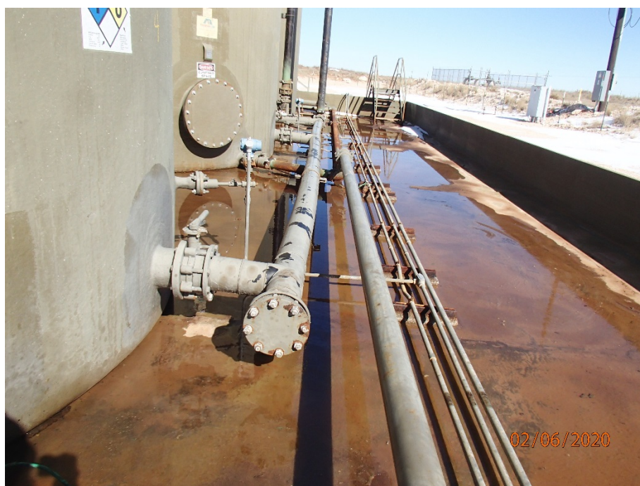
View showing the liner was almost completely filled with and holding precipitation.
