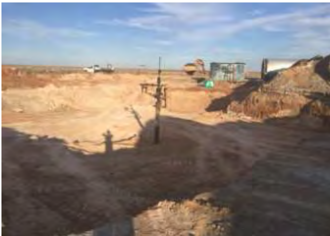
Photos 4 & 5: Post excavation of wellhead area
