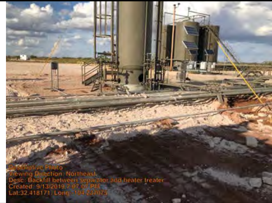
Backfill between separator and heater treater
