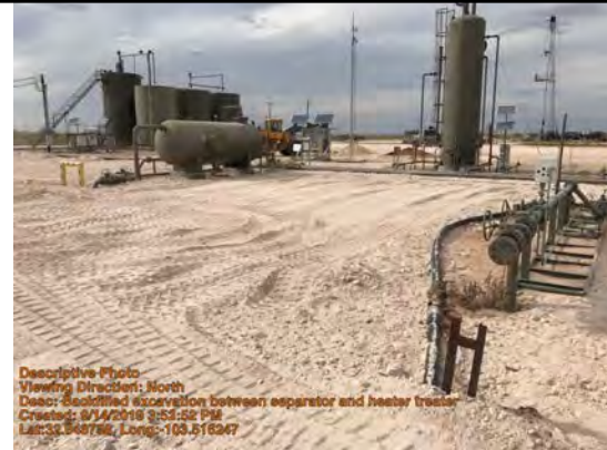
Backfilled excavation between separator and heater treater
