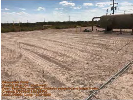
Backfilled excavation between separator and heater treater
