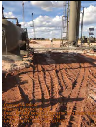
Backfill between separator and heater treater
