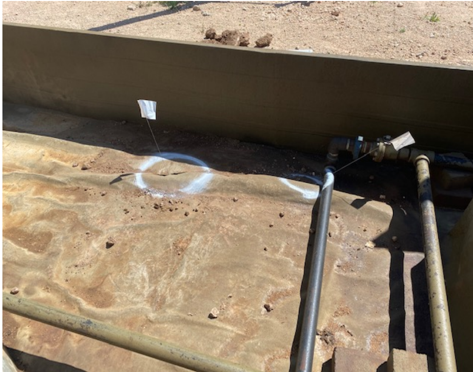
Photograph 1: View of BH01 location along with secondary tear in liner.
