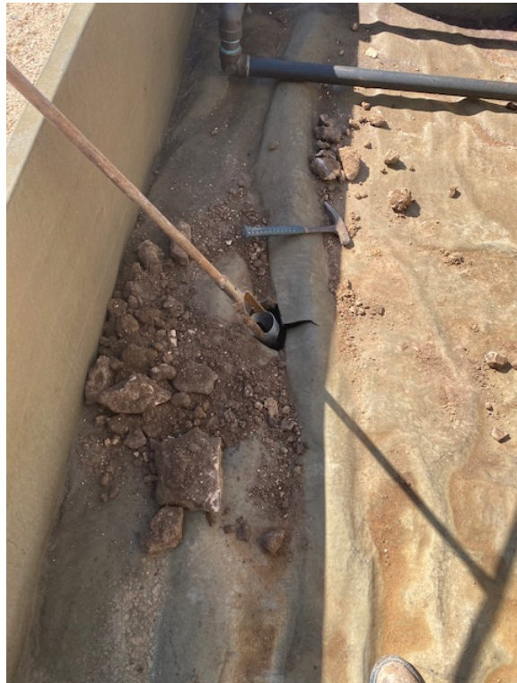
Photograph 2: BH01 location backfilled and the liner was repaired.
