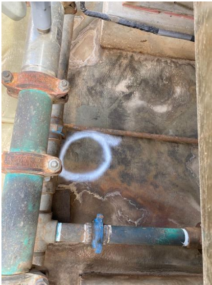
Photograph 3: View of liner tear
