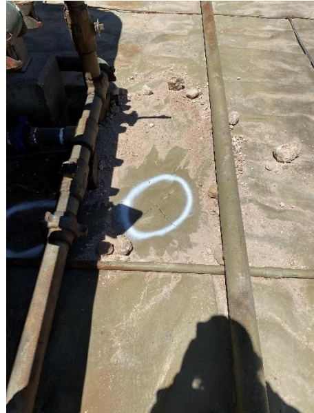
Photograph 4: View of backfilled bore hole through liner
