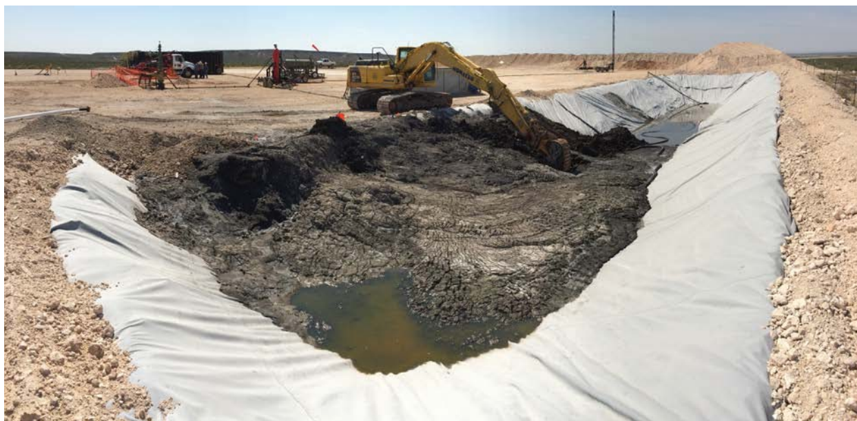
Figure 2 – Photo shows excavation of the second of five sampling trenches. A representative sample of each trench was extracted by scraping the edge of each trench with the bucket. The material was piled on the edge of the pit and Mr. Hicks obtained two composite/representative samples from each pile and placed them in an orange or blue 5-gallon bucket. The final composite sample was a mixture of each bucket.
