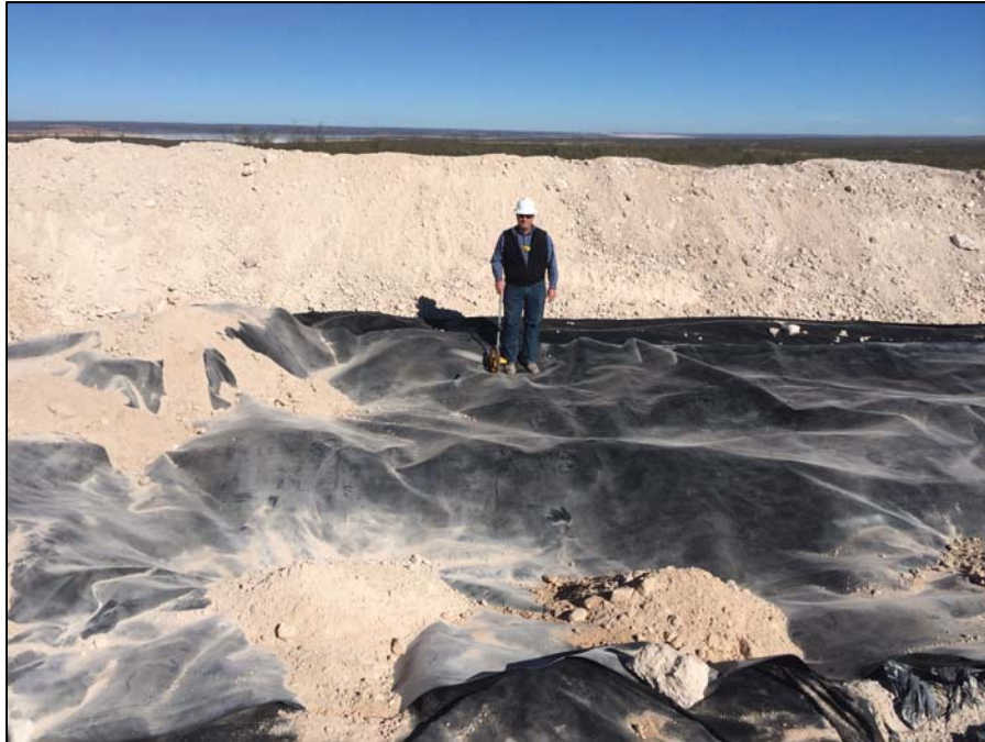
Geomembrane cover over stabilized cuttings >4 ft below grade
