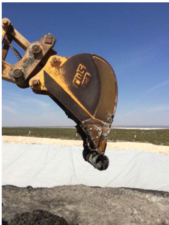
Figure 1 – Track hoe bucket with teeth covered by poly pipe to minimize the potential of ripping the liner.
