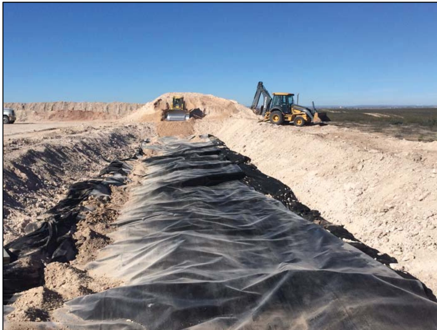
Backfilling over geomembrane cover; felt visible on edges of liner
