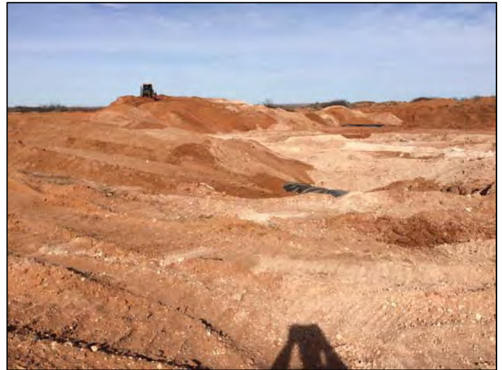
Backfilling over geomembrane liner 2/8/2017
