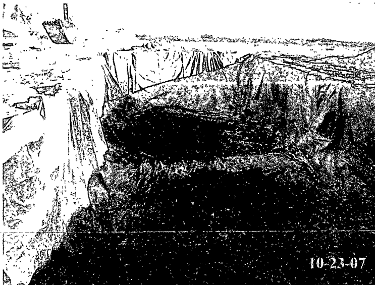
Burial pit lined with a 12 mil impervious liner.
