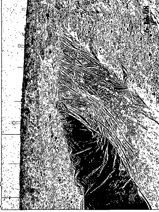
First burial pit lined with 12 mil poly liner.
