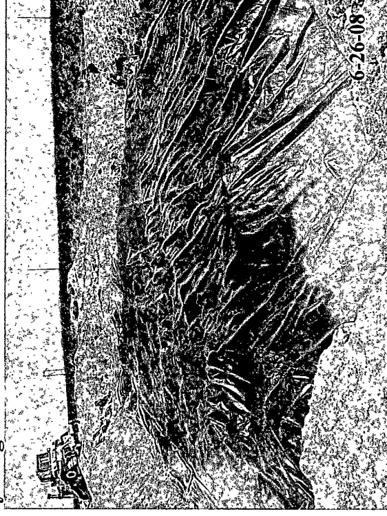
Second burial pit capped with 20 mil poly liner.
