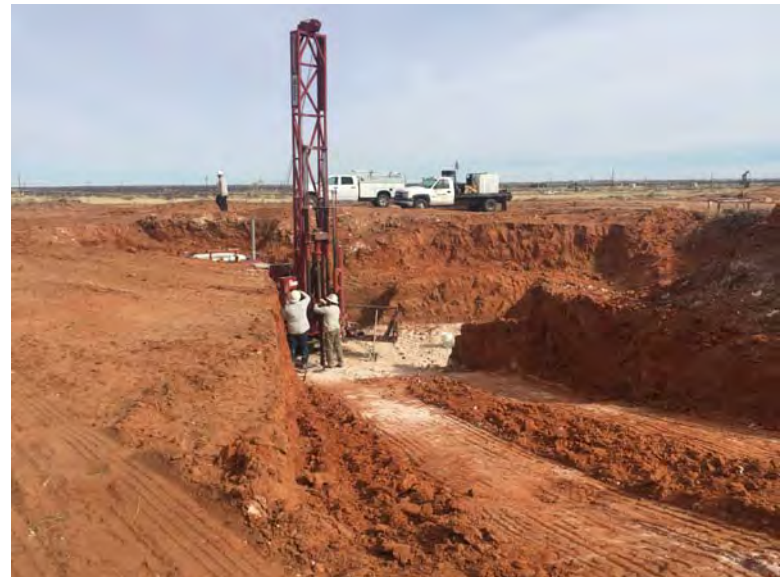
Photo #12 : View facing ENE showing hollow-stem drilling rig at 12 ft bgs on floor of vent excavation (01/17/2019)
