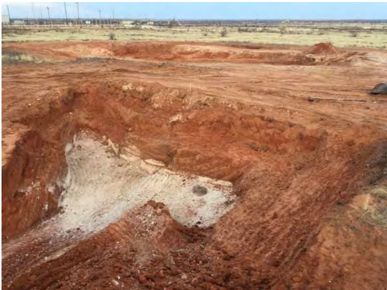
Photo #11 : Facing northeast showing completion of excavation to 12 ft bgs into caliche layer at vent area (1/10/2019)
