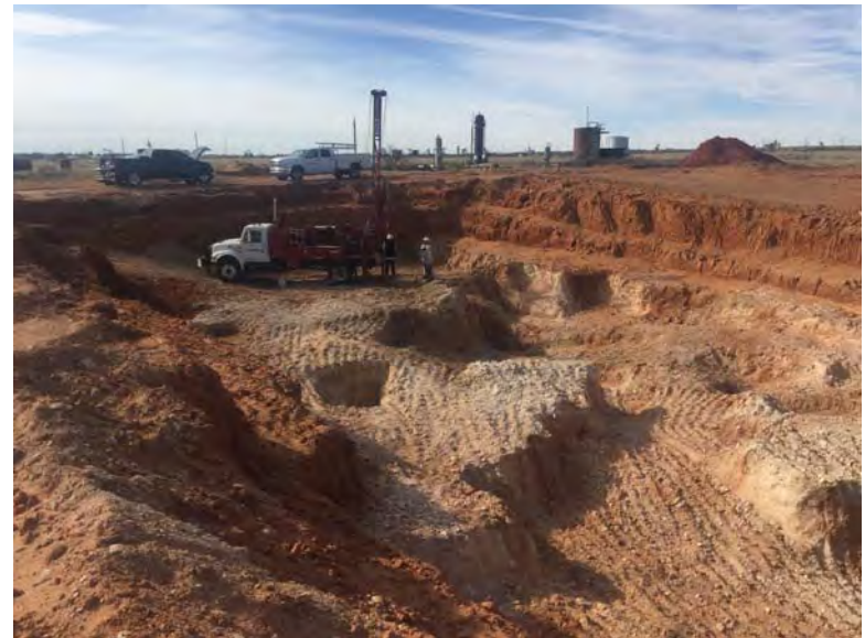
Photo #8: View facing southwest showing hollow-stem drilling rig at 15 ft bgs on floor of south end of pit area (01/17/2019)
