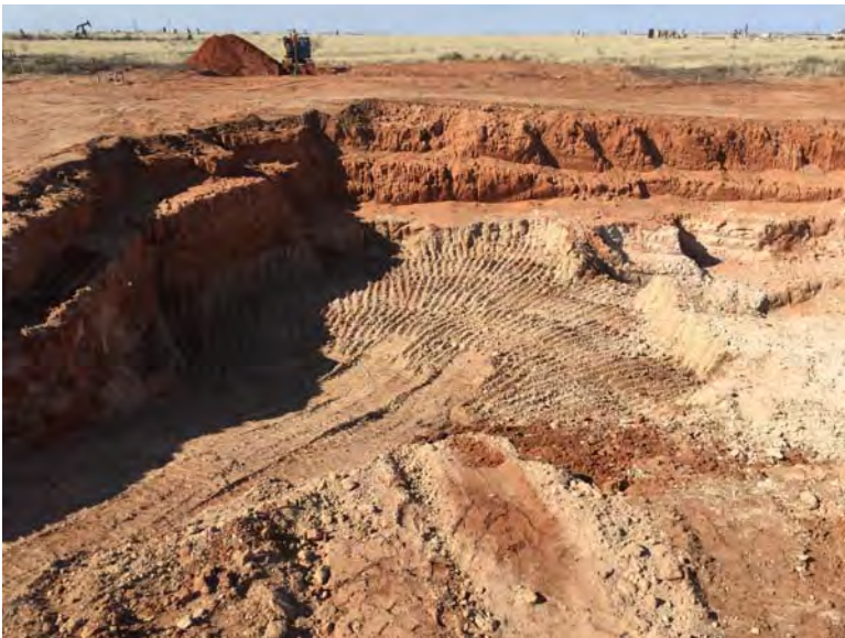
Photo #7: Facing WNW after 3 more ft of soil removed (15 ft bgs) at south end of pit area & ramp built for drilling access (1/10/2019)
