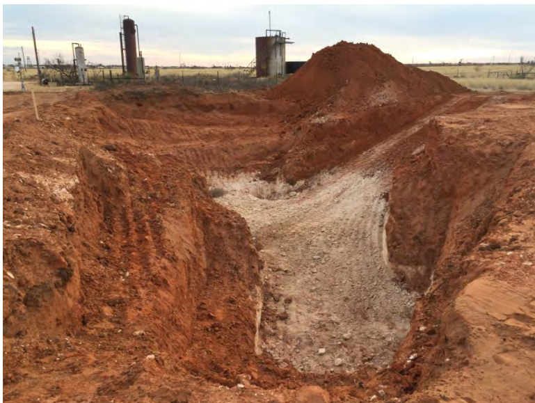
Photo #7 : Vent excavation facing south prior to chemical oxidation treatment (01/10/19)
