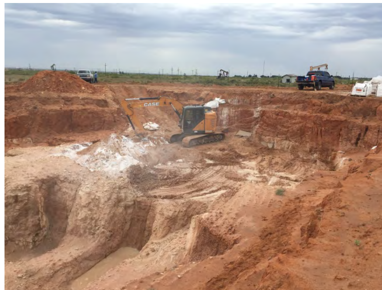
Photo #4: Dry-blending chemical oxidants (sodium persulfate and calcium hydroxide) into soil (grid P; 7/2/19)
