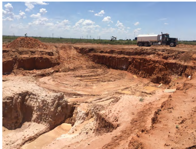
Photo #6 : Pit excavation facing southeast after completion of chemical oxidation treatment in grids M-N-O-P (7/2/19)
