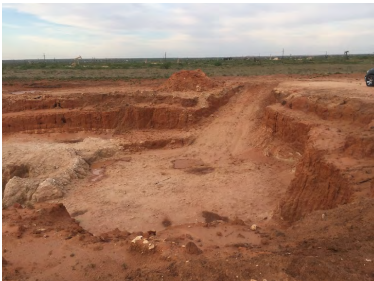
Photo #1: Pit excavation facing southeast prior to addition and mixing of chemical oxidants into grids M-N-O-P (7/1/19)
