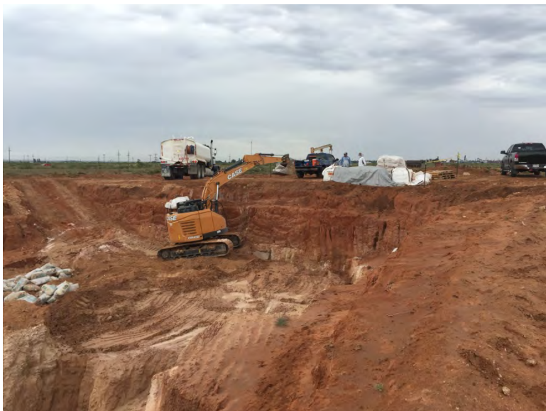
Photo #3: Adding calcium hydroxide on top of sodium persulfate prior to mixing into soil (grid P; 7/2/19)
