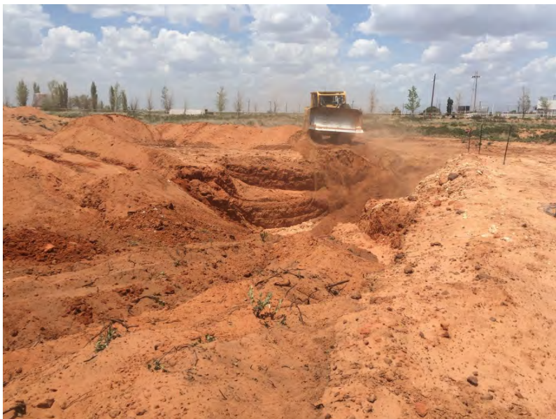
Photo #9: View facing northeast showing backfilling clean soil into vent excavation (7/31/19)
