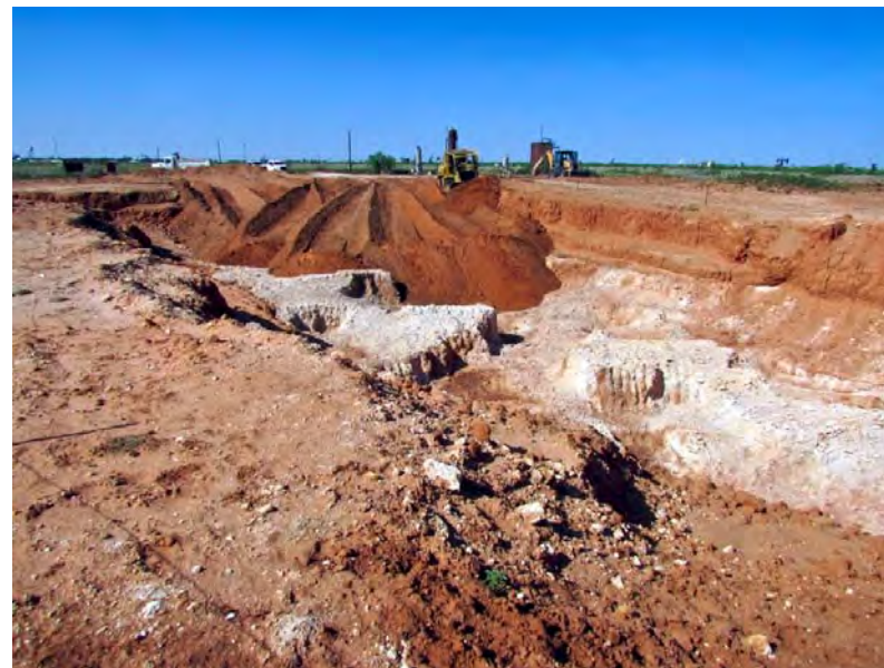
Photo #10: View facing southwest showing backfilling clean soil into pit excavation (8/1/19)
