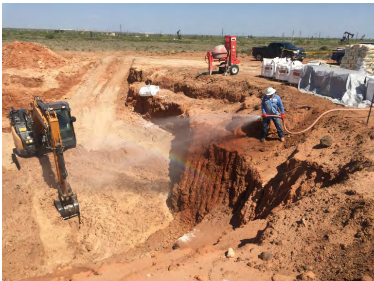
Photo #5 : Blending chemical oxidants (sodium persulfate and calcium hydroxide) and freshwater with soil (grid M; 7/1/19)
