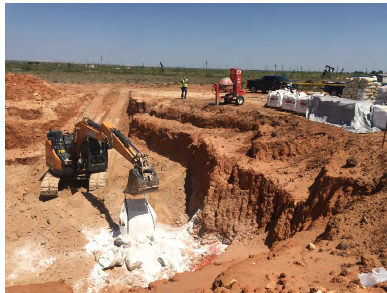
Photo #2: Addition of sodium persulfate into soil while still in dry state (grid M; 7/1/19)
