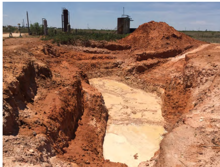
Photo #8 : View facing south at vent excavation after completion of chemical oxidation treatment (7/3/19)
