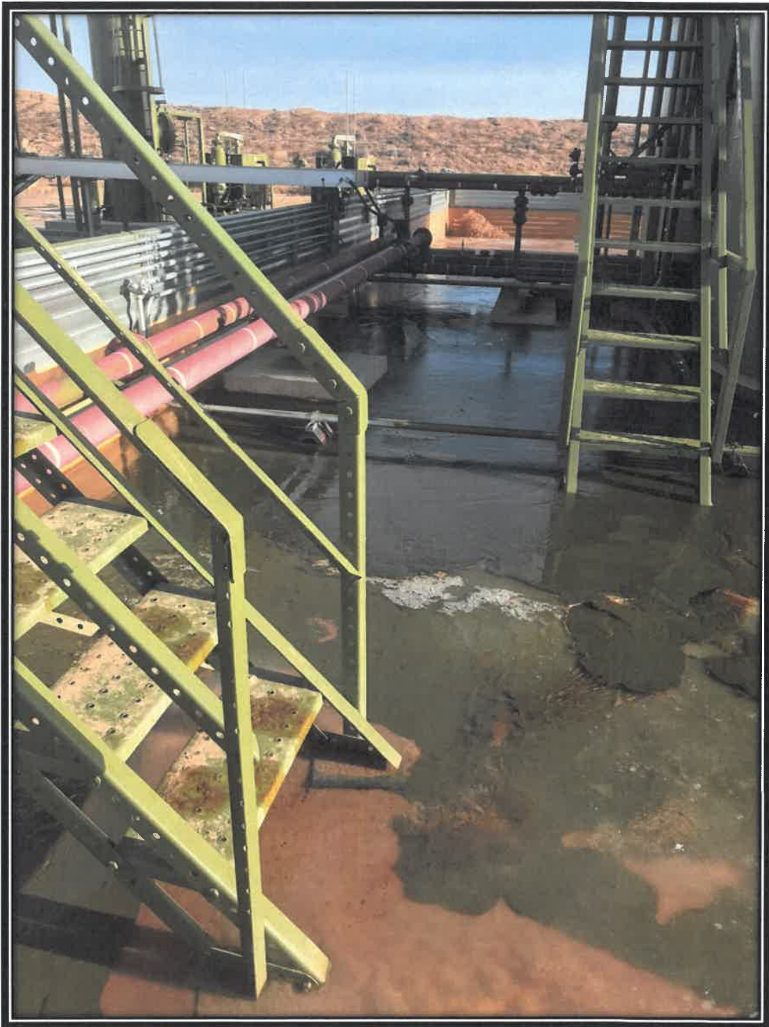
PHOTO 3: Oil Pooled in Lined Berm (View 2)
