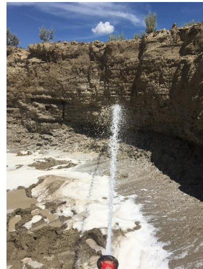
Photograph 12: Microblaze amendment application to cutbank.
