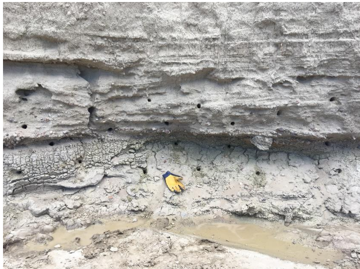
Photograph 11: Drill holes in cutbank prior to amendment application.
