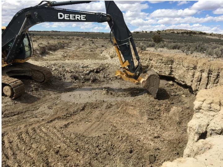
Photograph 5: Surface wash excavation between Dam 3A and 3B.
