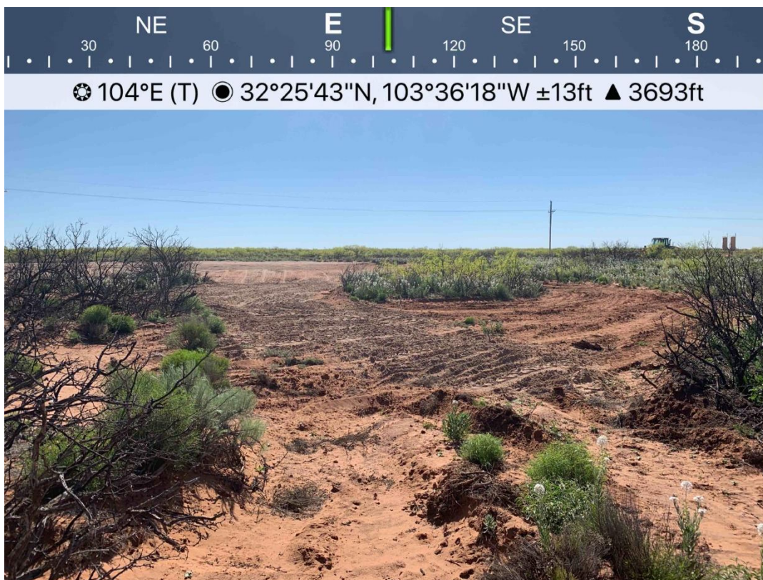
Backfilled and Seeded Area Viewing East, April 16, 2020
