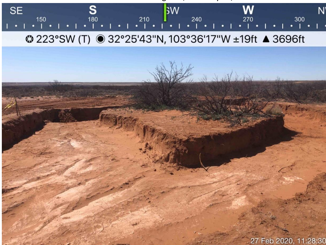
Excavation Area Viewing Southwest, February 27, 2020
