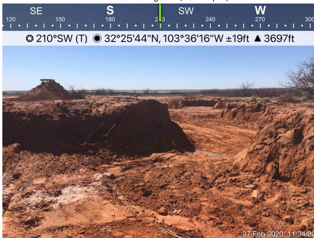
Excavation Area Viewing Southwest, February 27, 2020
