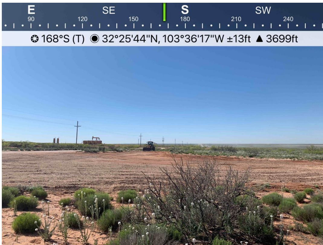
Backfilled and Seeded Area Viewing South, April 16, 2020
