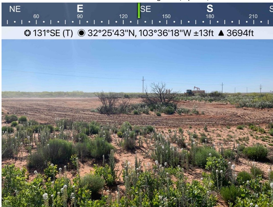
Backfilled and Seeded Area Viewing Southeast, April 16, 2020
