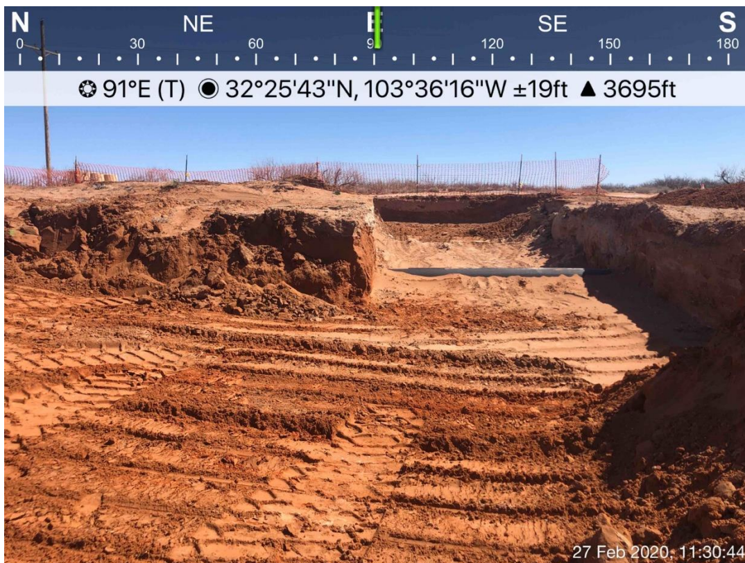
Excavation Area Viewing East, February 27, 2020
