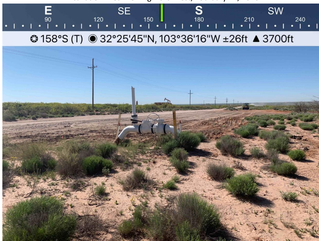
Backfilled and Seeded Area Viewing South, April 16, 2020
