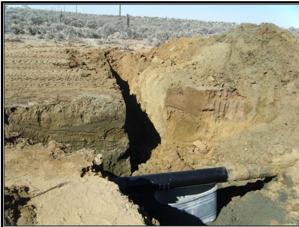
Photo 5: Trenching to Find Extent of Contamination
