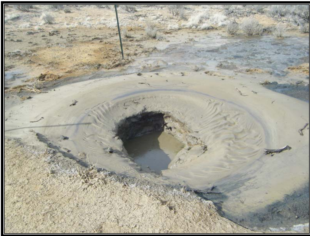
Photo 1: Pipeline Leak Breaking Ground Surface
