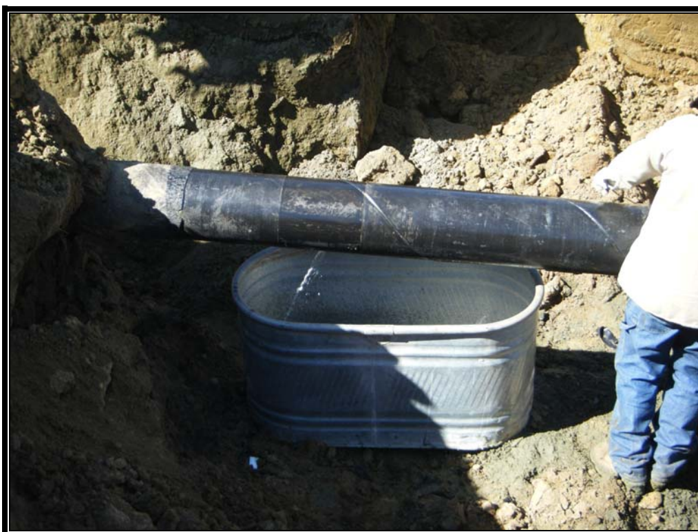
Photo 6: Leaking Pipeline
