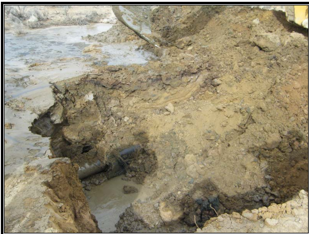
Photo 2: Exposing Leaking Pipeline
