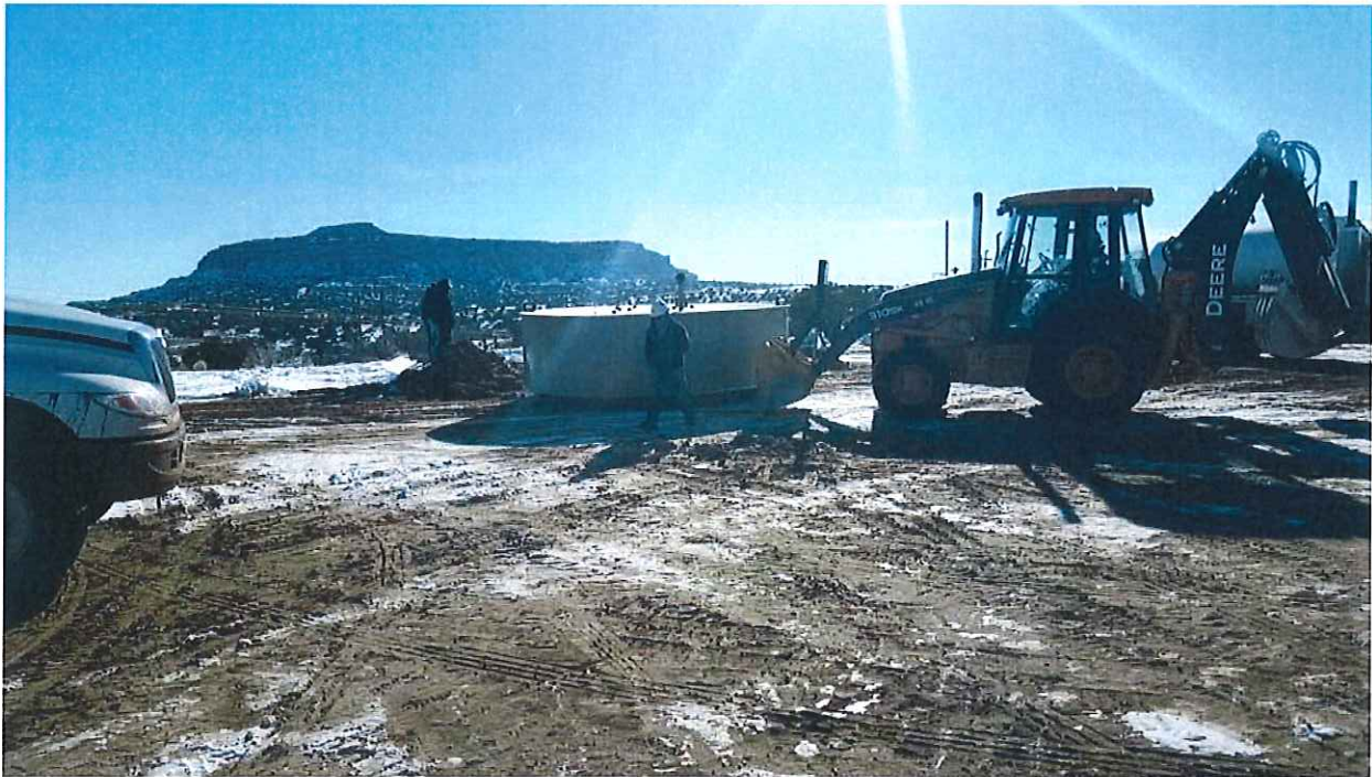
Photograph 1. View facing west-southwest of below grade tank following removal from the excavation.
