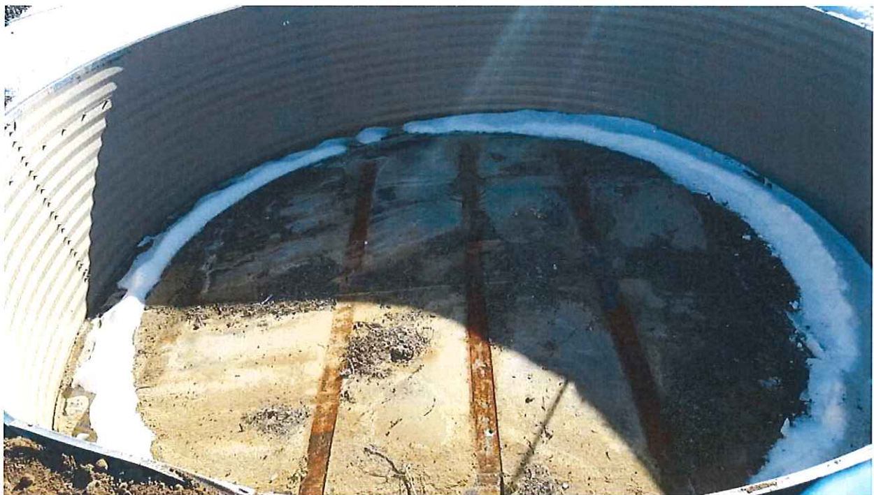
Photograph 2. View of liner in place following lifting the tank from the excavation.
