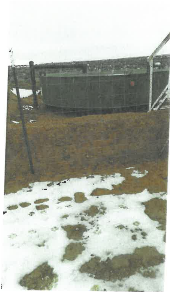
Photo 7: New above ground tank installed in the same location of the former BGT. Photo taken January 14, 2019.
