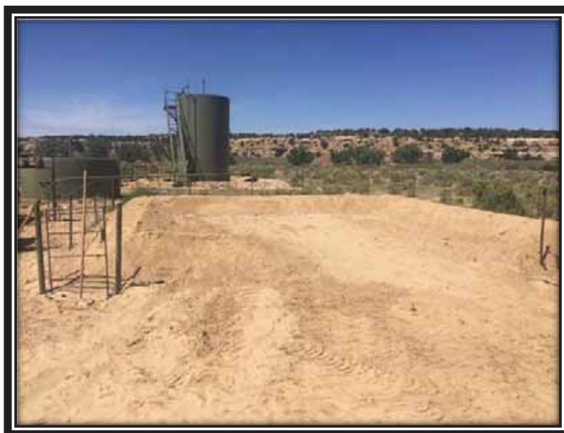
Picture 5: Subsequent Backfill of Release Site
